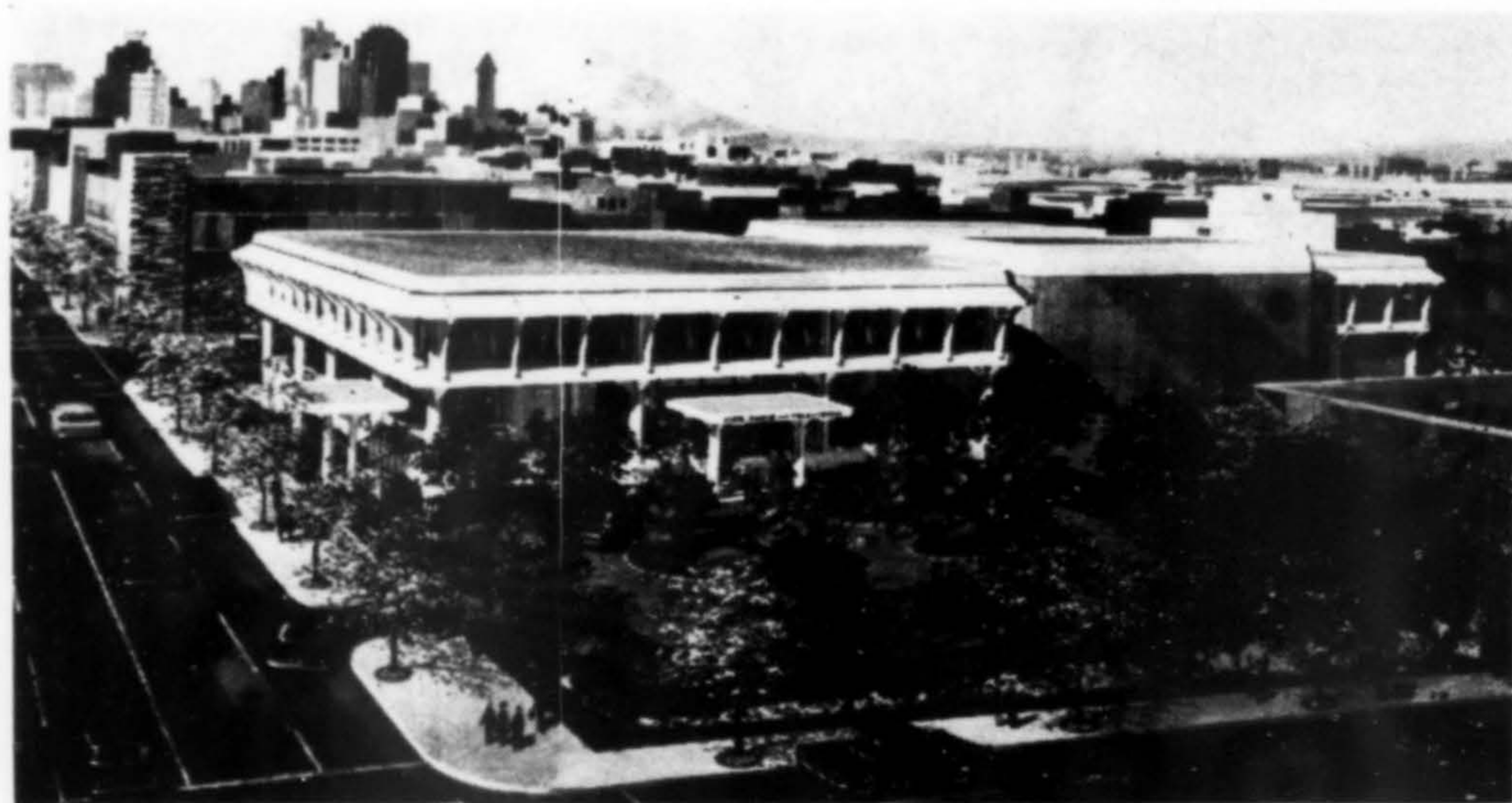
Broadcast House, now under construction in Seattle, will house KIRO-TV, KIRO-AM and KIRO-FM. The site, three-quarters of a city block, is near the Seattle Center. The two-story structure is designed to accommodate a future third floor of 12,000 sq. ft. One-third of the site has been developed as a landscaped drive-in entry creating a park-like setting. The multi-million dollar facility was designed by Fred Bassetti & Company, architects, with J. William Dimmich, partner in charge. Howard S. Wright Construction Co. is general contractor.
