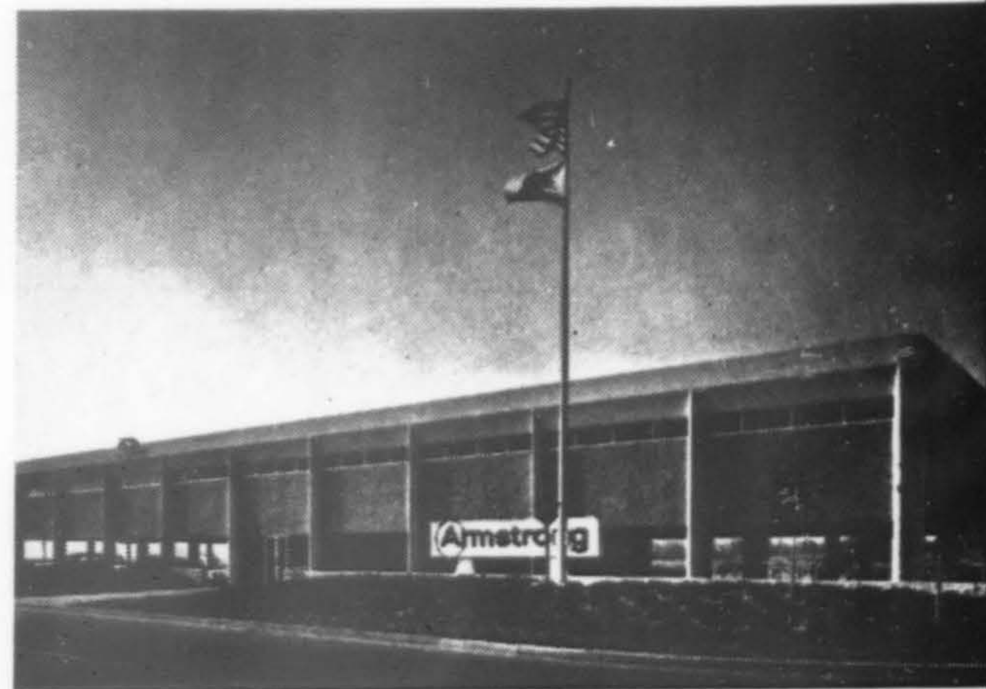
ARMSTRONG CORK COMPANY's new Los Angeles district office building at the Gilbert-Flair Industrial Park, El Monte, is headquarters for regional offices of four of the firm's marketing divisions. The building, a reinforced concrete structure, was designed by architects Langdon & Wilson. The William W. Gee Construction Company was general contractor.
