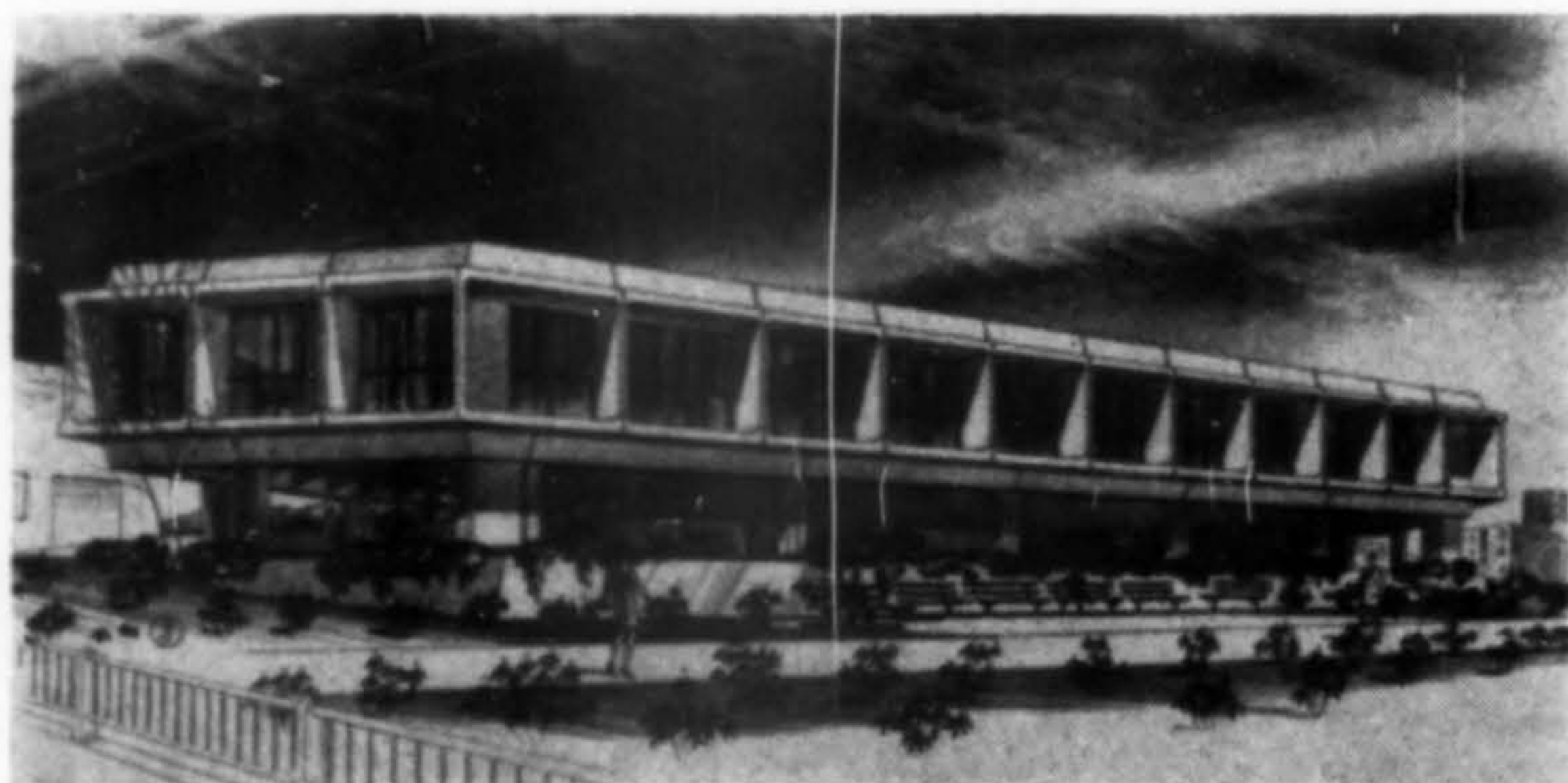
OFFICE BUILDING for University Properties, Seattle, will have Olivetti-Underwood as prime tenant. The $150,000 structure (8,000 sq. ft.) of precast and poured concrete will rise over surface parking for 26 cars. Architect: Richard Bouillon, AIA, & Associates; Olsen and Ratti, structural engineer.
