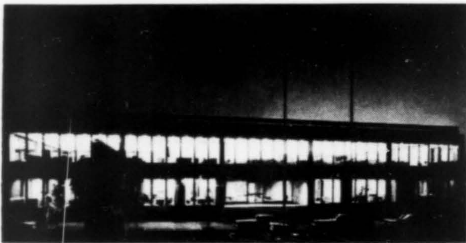
OFFICE BUILDING , Esco Corporation, Portland, Oregon. Wolff-Zimmer-Gunsul-Frasca, architects; Cooper & Rose & Associates, structural engineer; Henry M. Mason Company, contractor; Fought & Co., Inc., steel fabricator.
