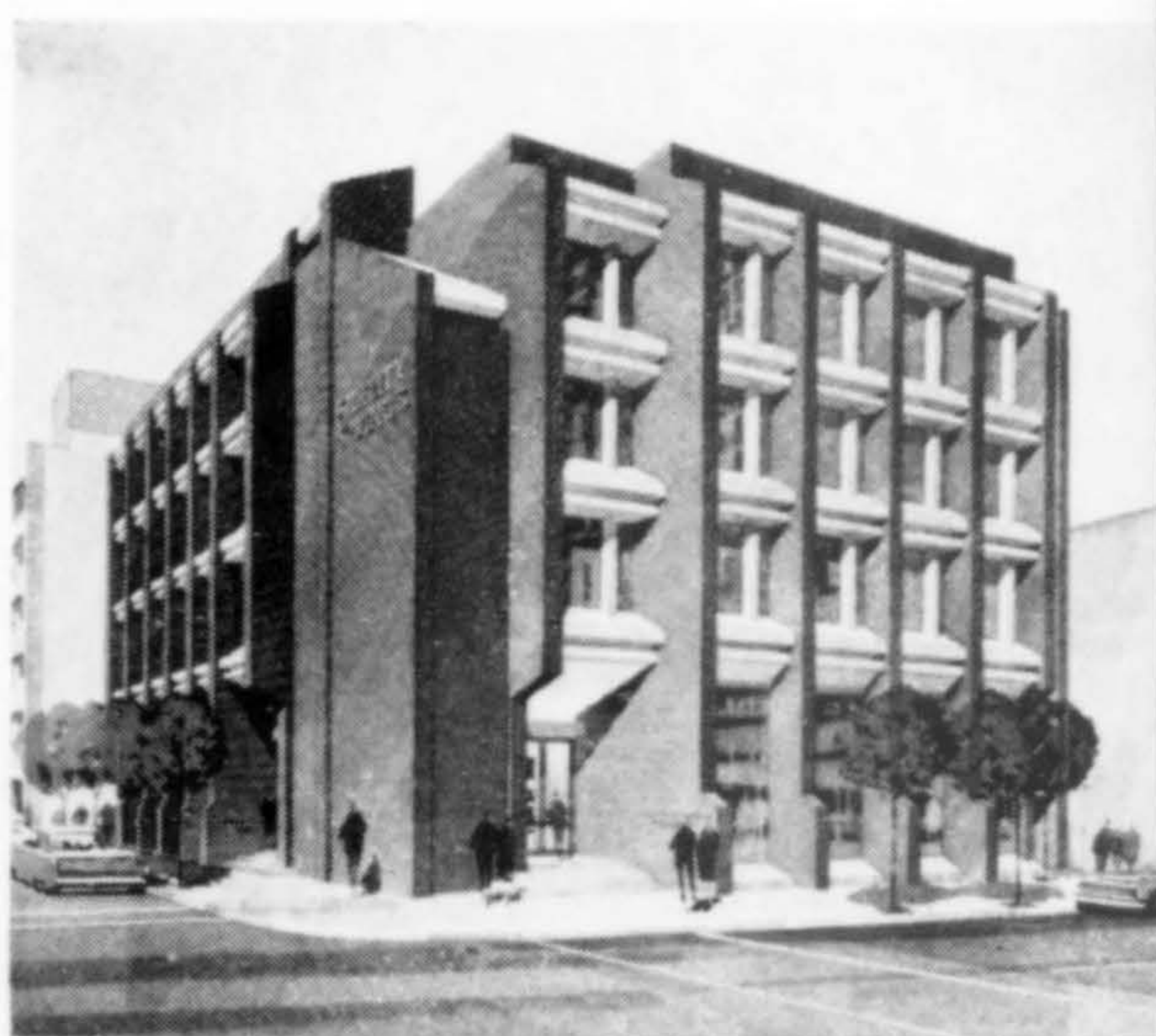
Fidelity Savings & Loan Association office building, Oakland, is new regional headquarters for the association. The brick structure features a series of full height vertical brick masonry piers along the two street fronts. Cost: $1,000,000. Architect: Robert Goetz Associates.
