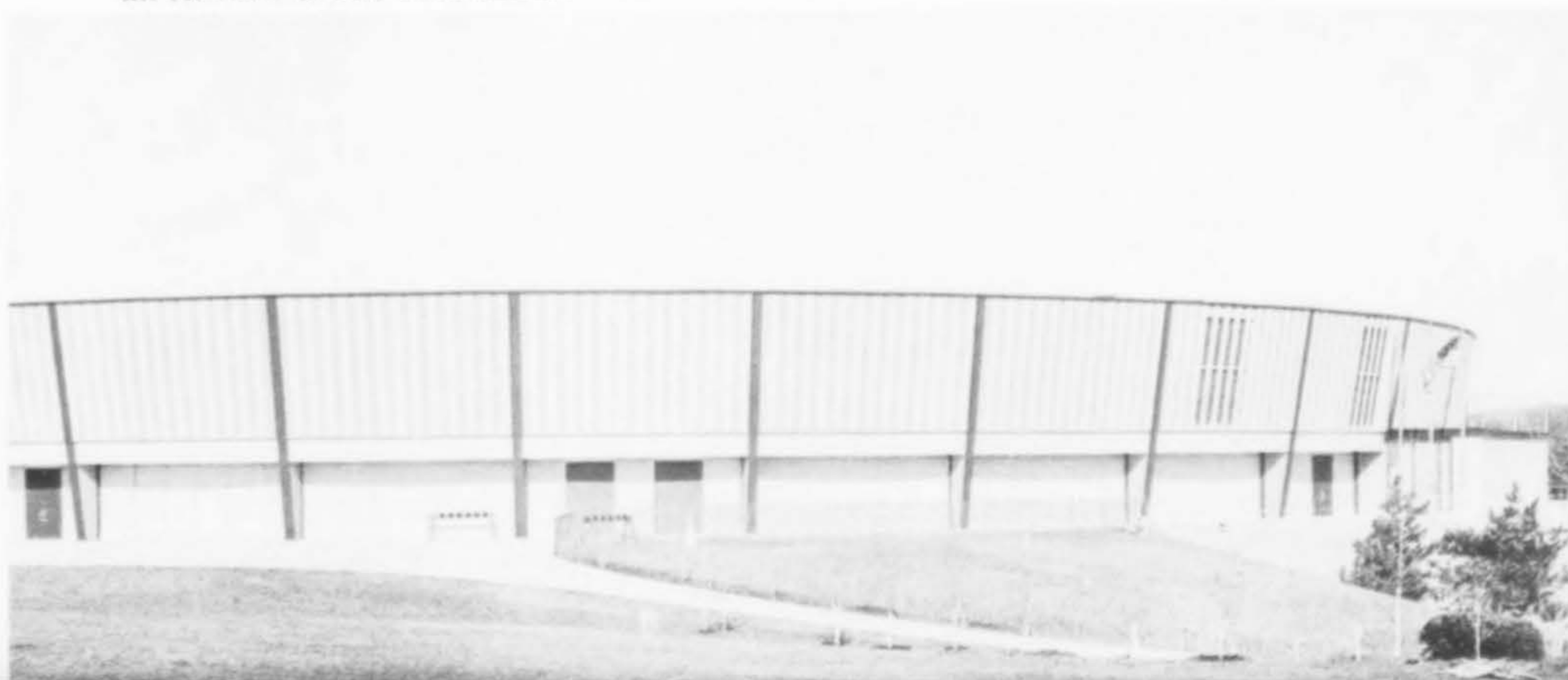
BELOW—THE PHYSICAL EDUCATION AND MILITARY TRAINING BUILDING at Southern Illinois University, Carbondale, Ill.; The Perkins & Will Partnership, Architects; M. H. Wolf & Co., Contractor.
