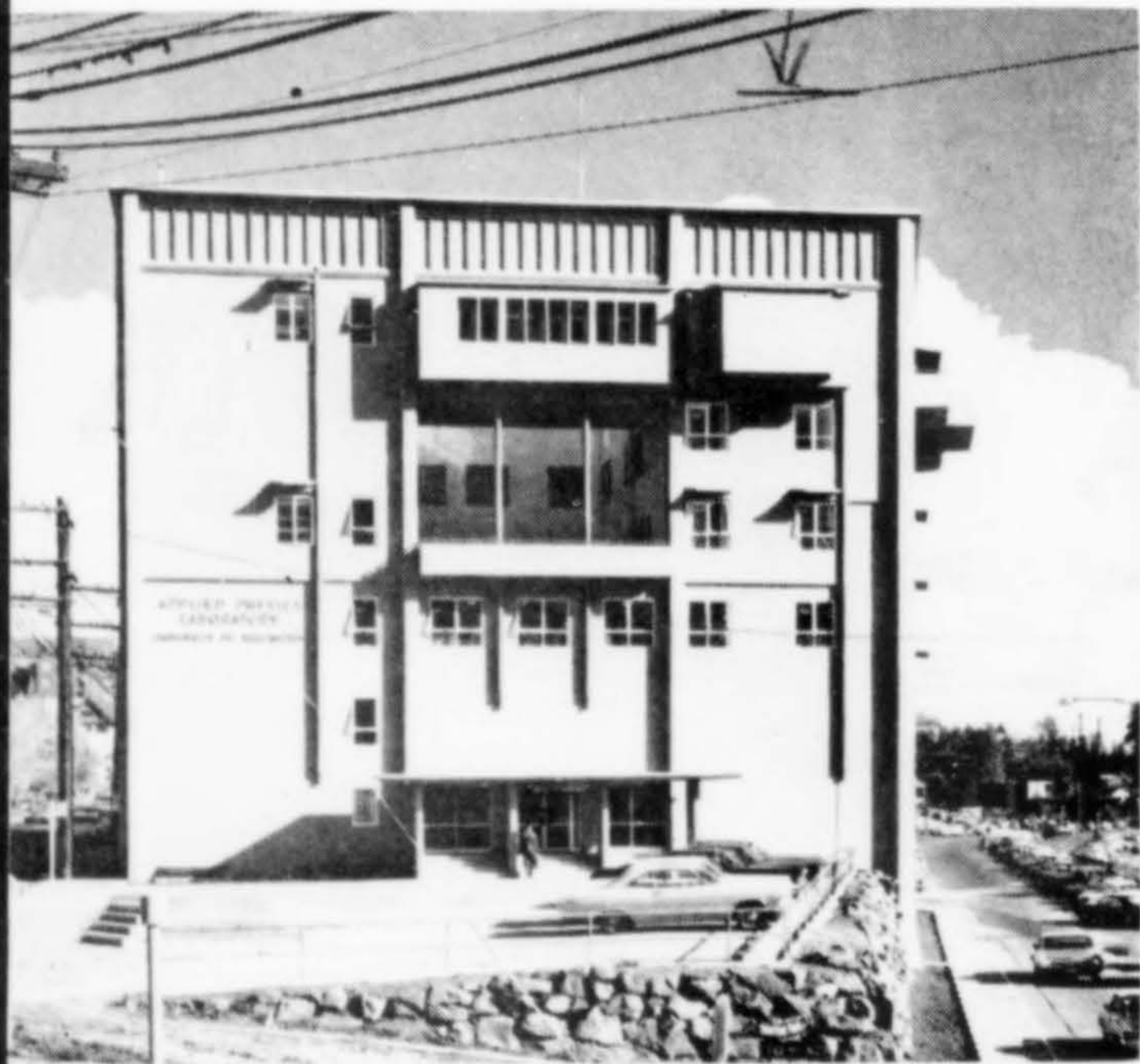
ADDITIONS and ALTERATIONS at the Applied Physics Laboratory, University of Washington. Honor Award. A. O. Bumgardner & Partners, architect.
