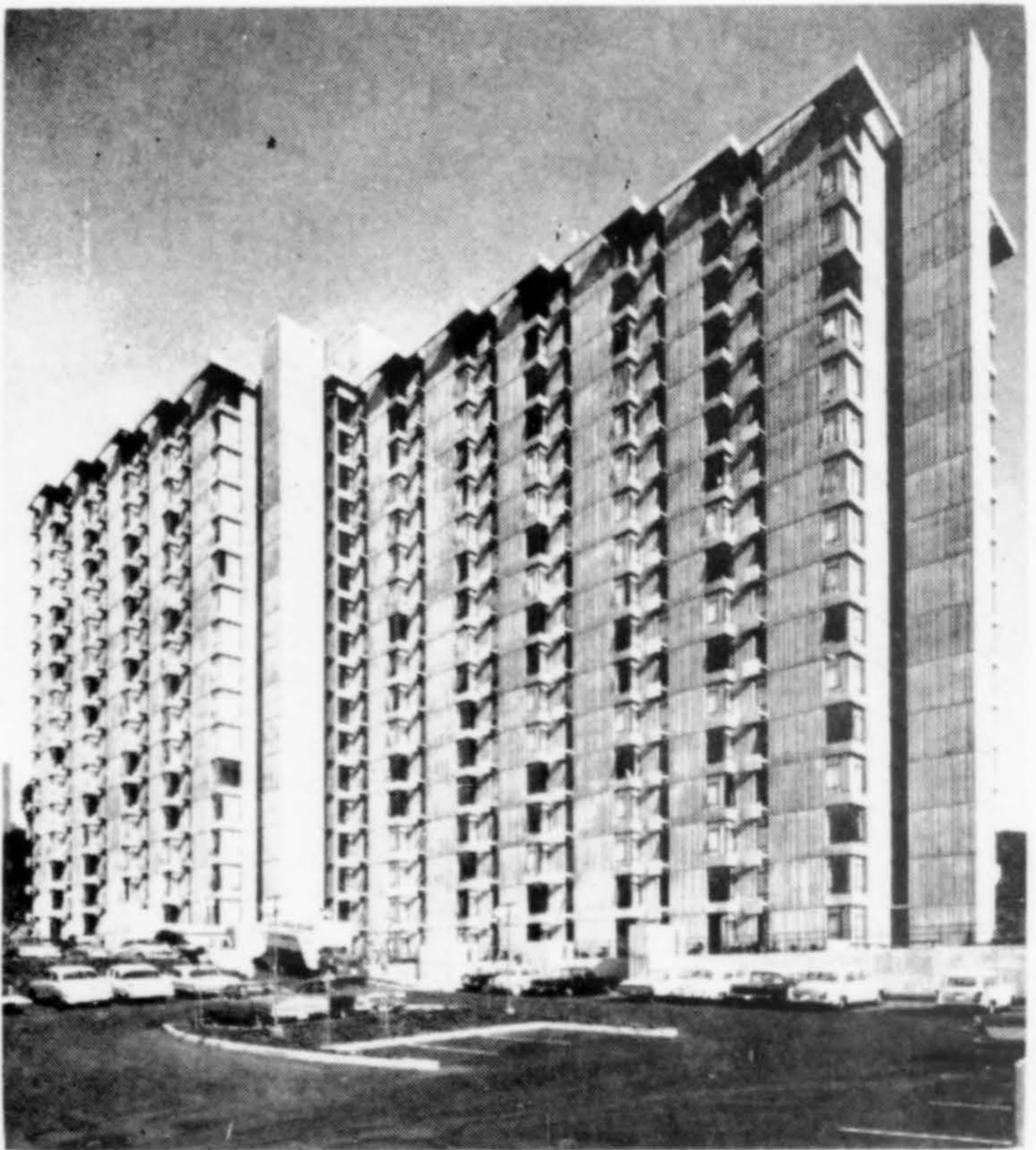
JEFFERSON TERRACE Apartments for the Elderly, Seattle Housing Authority, Seattle. Honor Award. Kirk, Wallace, McKinley & Associates, architect. (A/W, February 1968)
