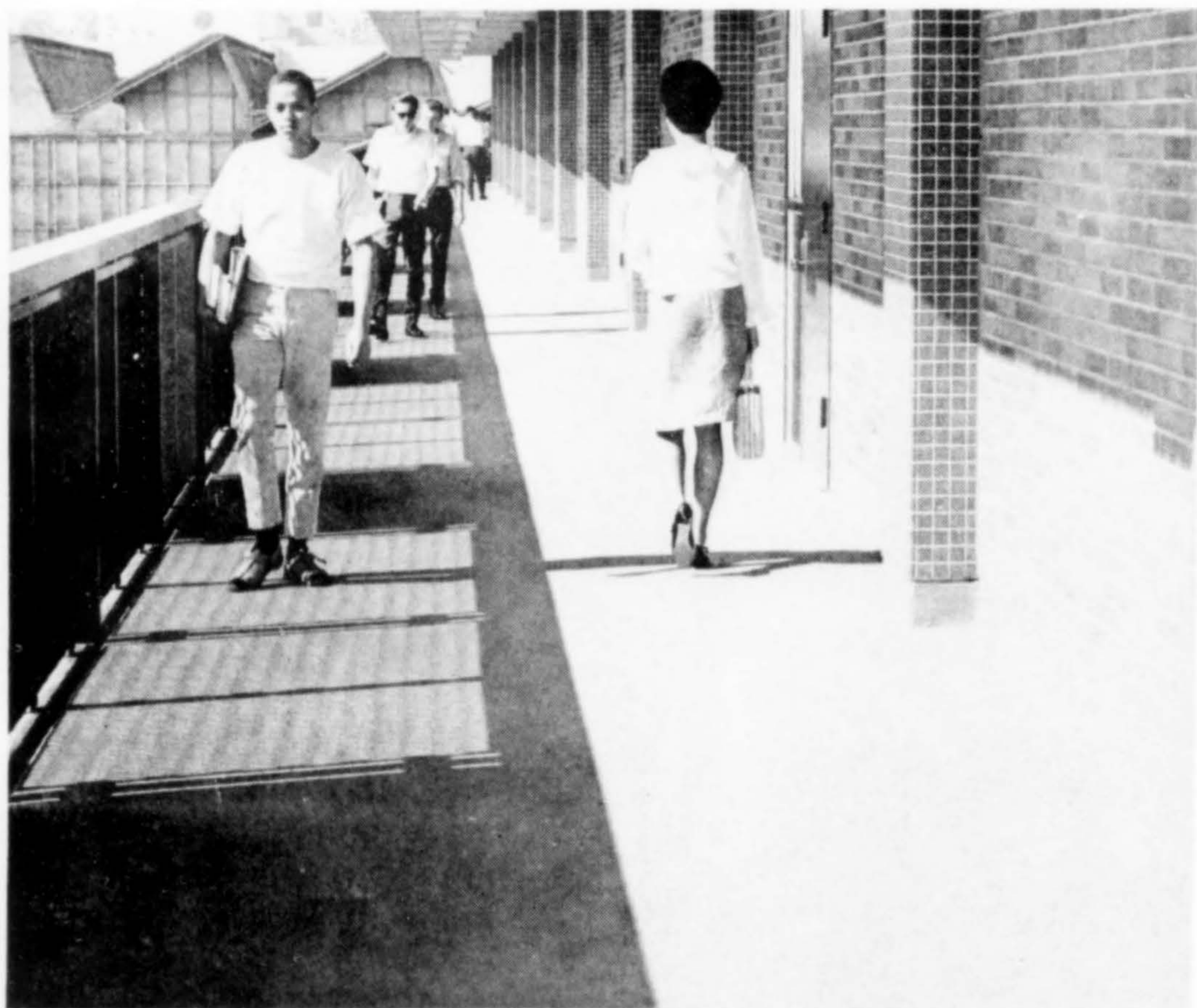
Technology Bldg., Pasadena City College, Pasadena, Calif. Architects: Allison & Ribbe, Applicator: Owen Roofing Co., Los Angeles.
