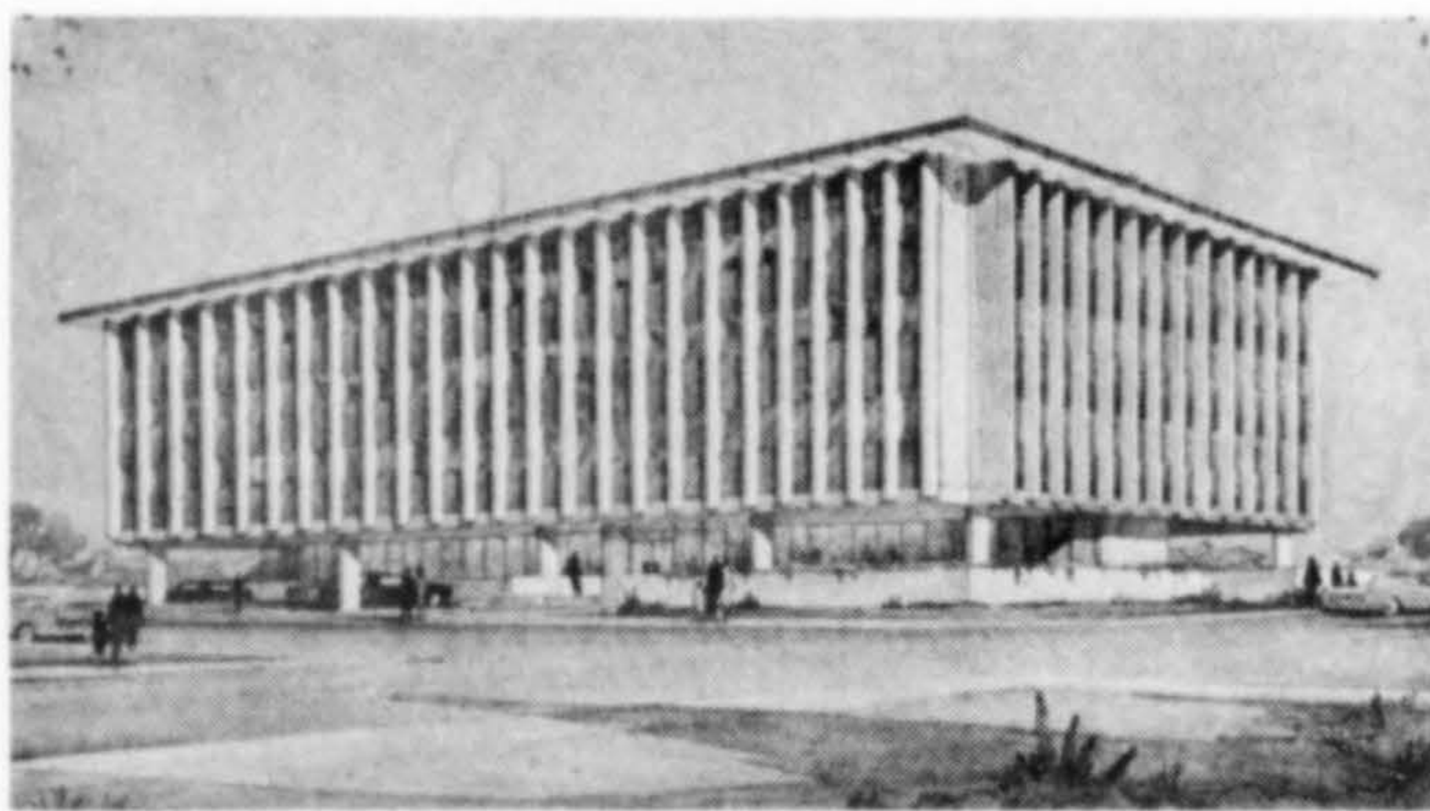
MEDICAL BUILDING , Reno, Nevada, will accommodate 25 doctors and related facilities. The structure has a cast-in-place concrete frame with precast concrete fins on the facades. Cost: $1.2 million. Architect: Hewitt C. Wells; Jacobsen Construction Co., Inc., contractor.
