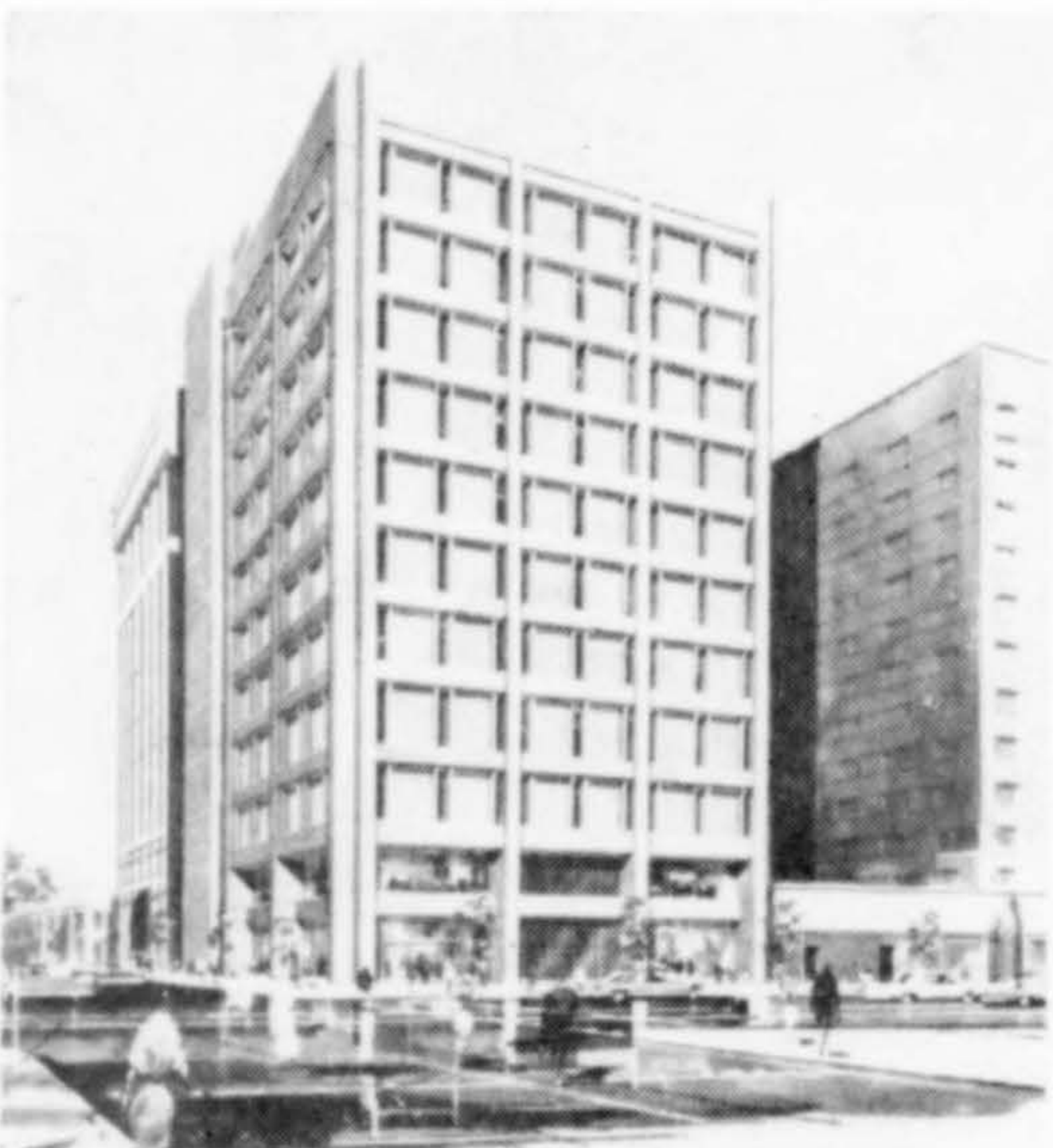
COMMUNICATIONS COMPLEX for Pacific Northwest Bell Telephone, Portland, will be reinforced concrete with precast facing units. The 11-story building will house latest in space-age equipment. Total cost: $10 million. Completion: January 1970. Architect: Wilmsen, Endicott & Associates.
