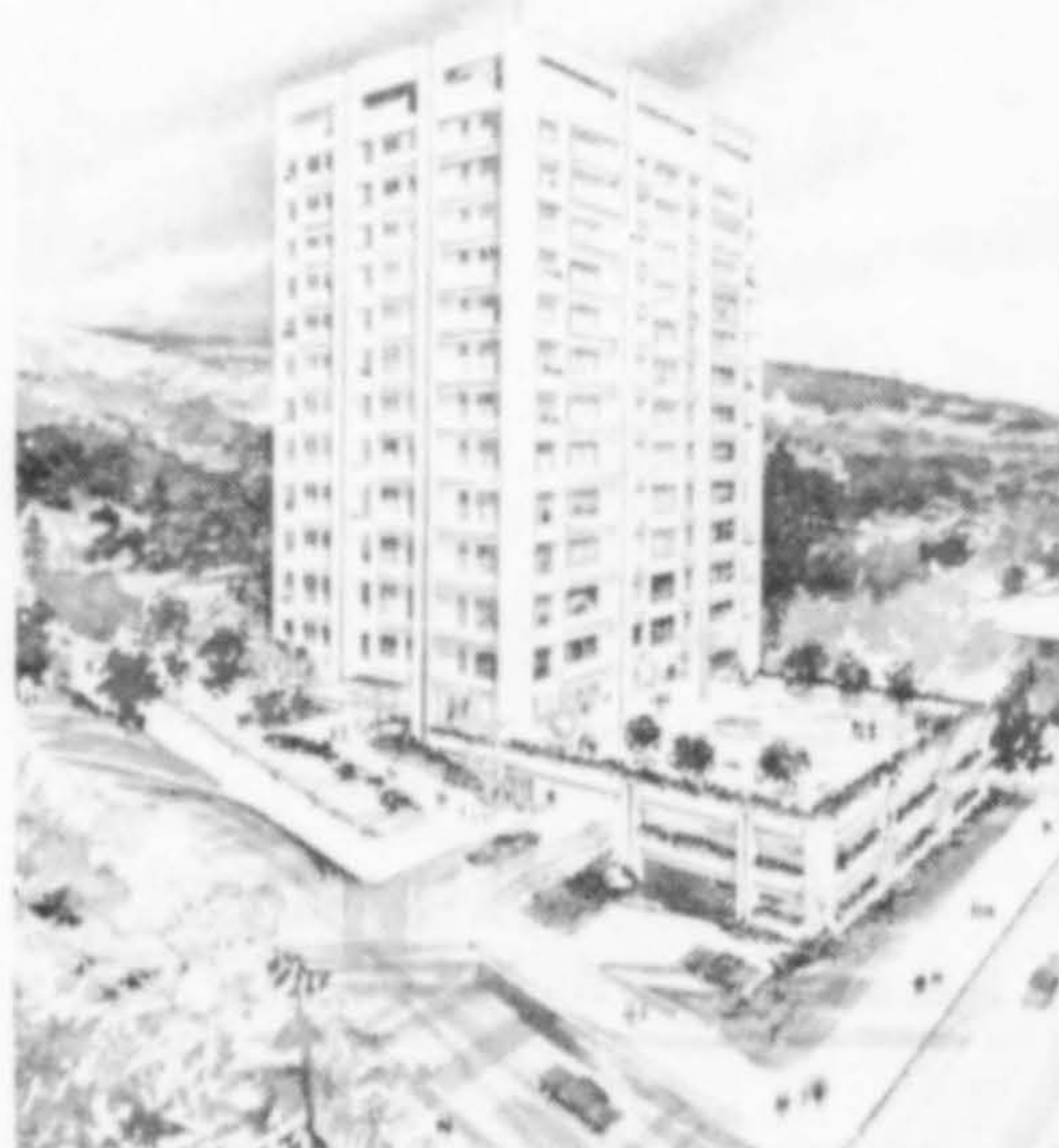
ALKI-BONAIR Retirement Community Center, Seattle, will be 16 stories with 86 units. The structure will be reinforced concrete with precast concrete exterior walls. Outdoor terrace and multi-purpose rooms at third-floor level. Completion: early 1970. Cost: $1.94 million. Architect: Shavey & Schmidt.
