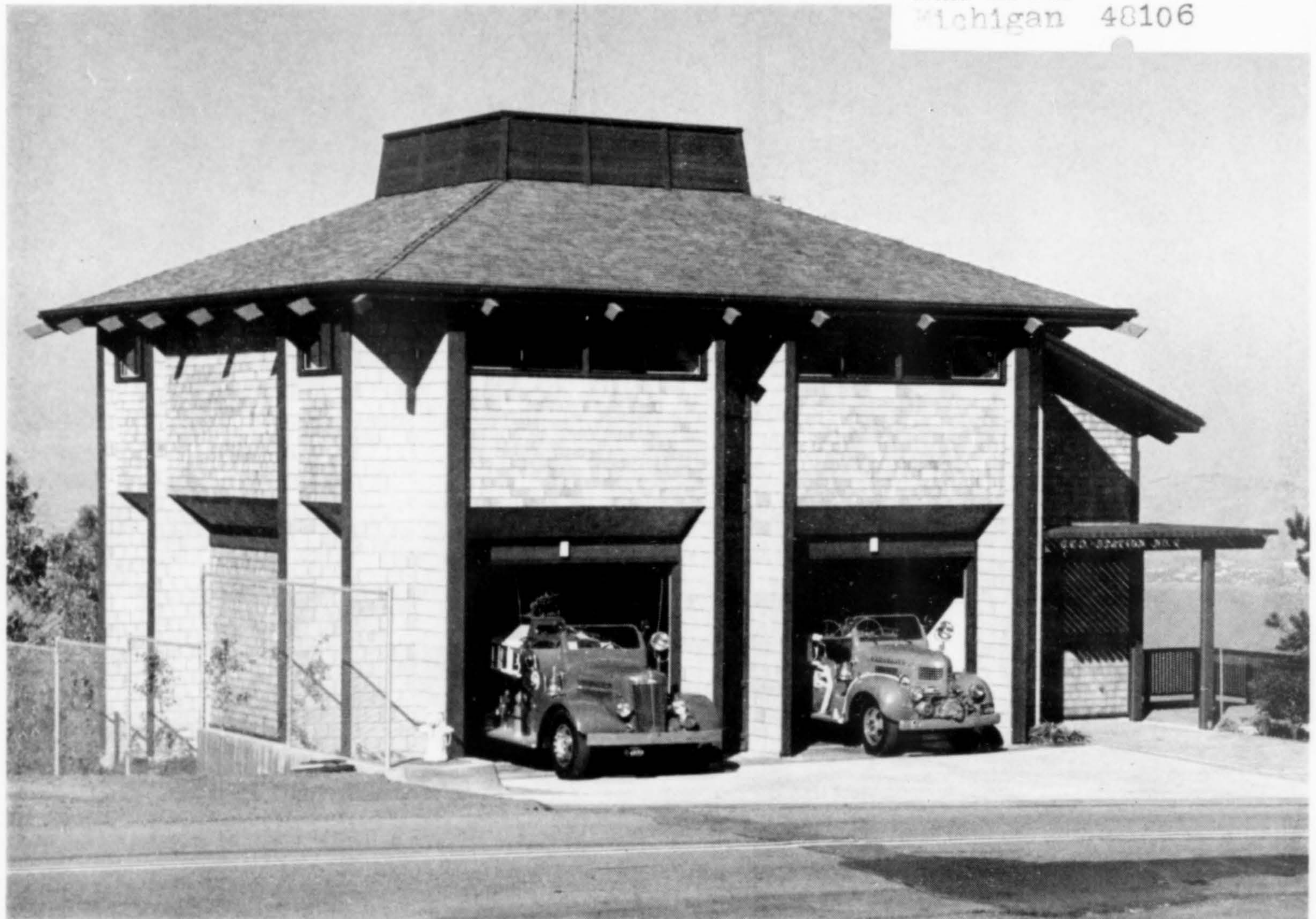
Fire station—Sausalito, California Architects: Rockne and Watson
