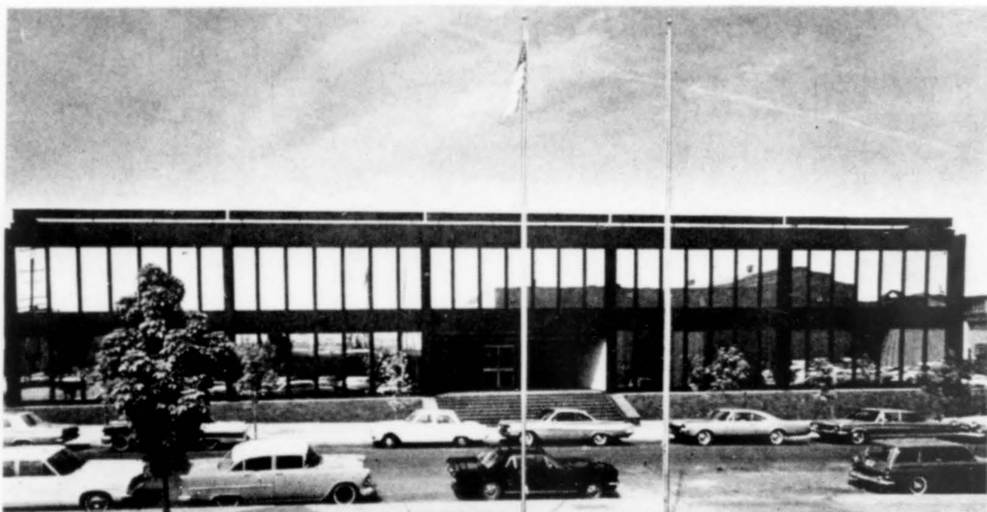
ADMINISTRATION BUILDING. ESCO Corporation. Honor Award. Architect: Wolff, Zimmer, Gunsul, Frasca & Ritter.
