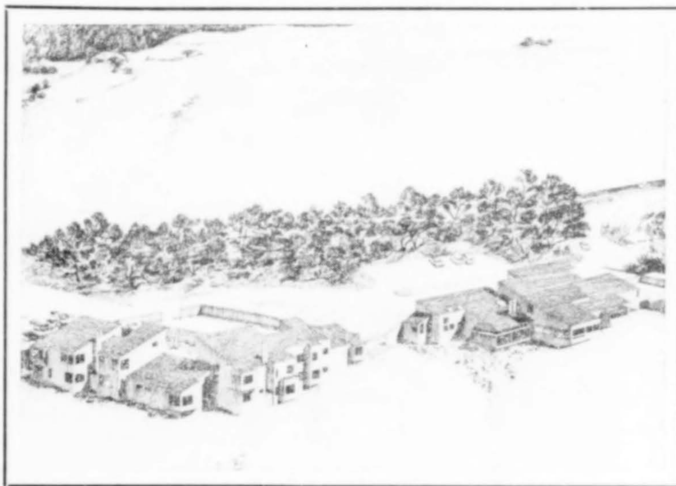
TWENTY-UNIT LODGE at The Sea Ranch on the Sonoma Coast, California, follows closely in design the pattern established by MLTW's and Esherick's condominium structure, store-restaurant nationally published. The lodge continues its reliance on woods of the area—redwood, cedar and fir. In shape, it forms an irregular "L" with an elongated western porch extending along the face of the complex. Architect was Sea Ranch's Planning Director, Louis McLane, AIA; with Agora Architects as associates; Lawrence Halprin & Associates, landscape.
