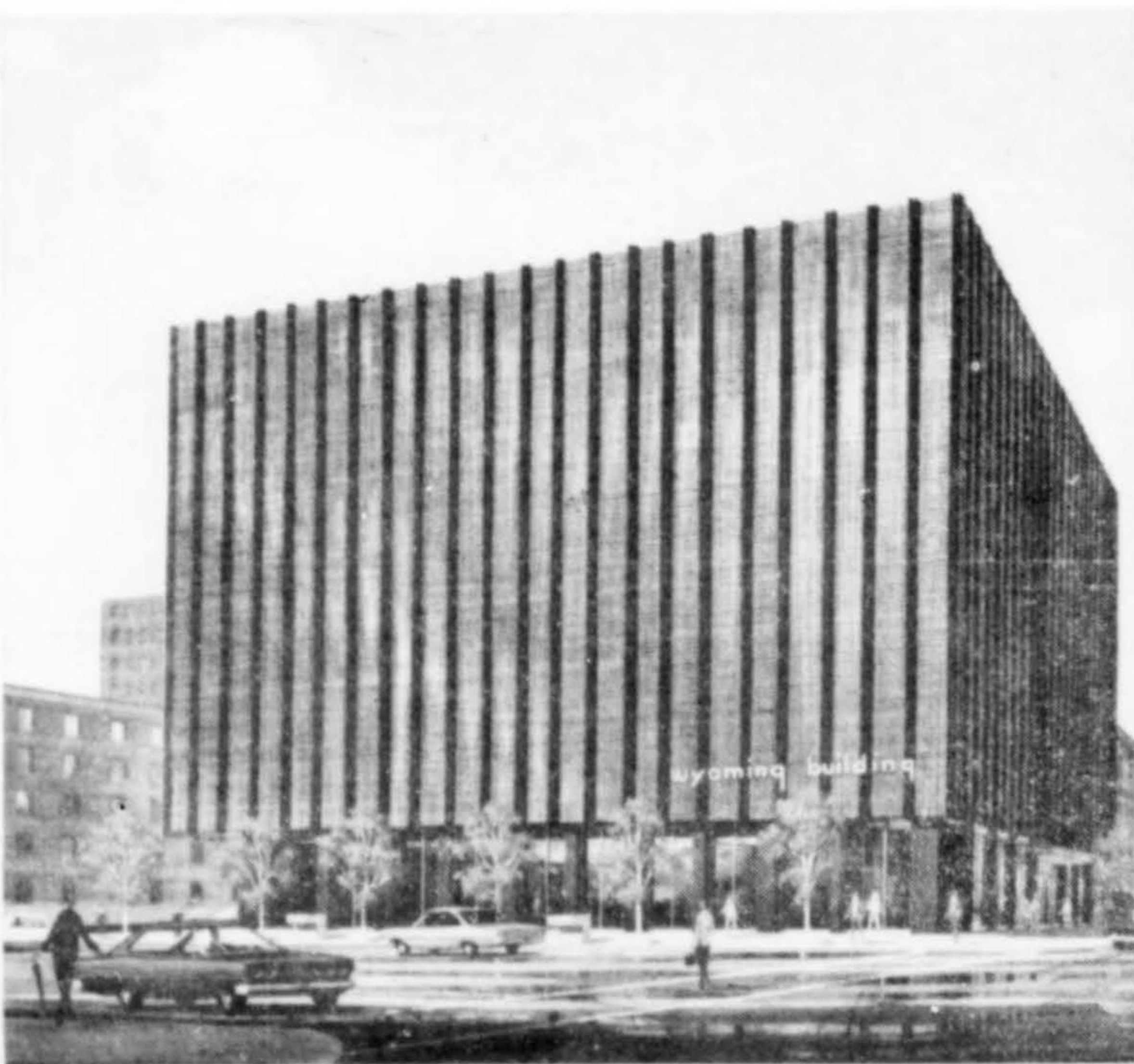
REMODEL OF WYOMING BUILDING , a 50-year-old structure, into offices for Pacific Power & Light Company, Casper, Wyoming. The building, due for completion in January, will be made "new" with a sun screen suspended away from the building. All stone work will be removed and one-inch L.O.F. thermopane installed, floor-to-ceiling, at exterior walls. Architect: Gerald Deines; Volk & Harrison, structural.
