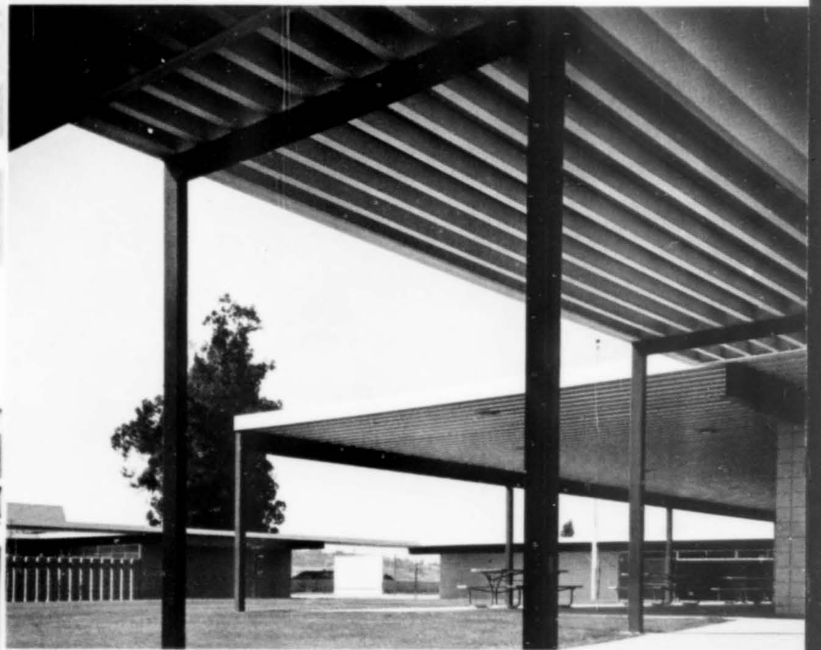
L S DECK—MADERA ELEMENTARY SCHOOL, Simi Valley, Cal.; Daniel, Mann, Johnson & Mendenhall, Archts. and Engrs.; Packard Constr. Co., Contractor.
