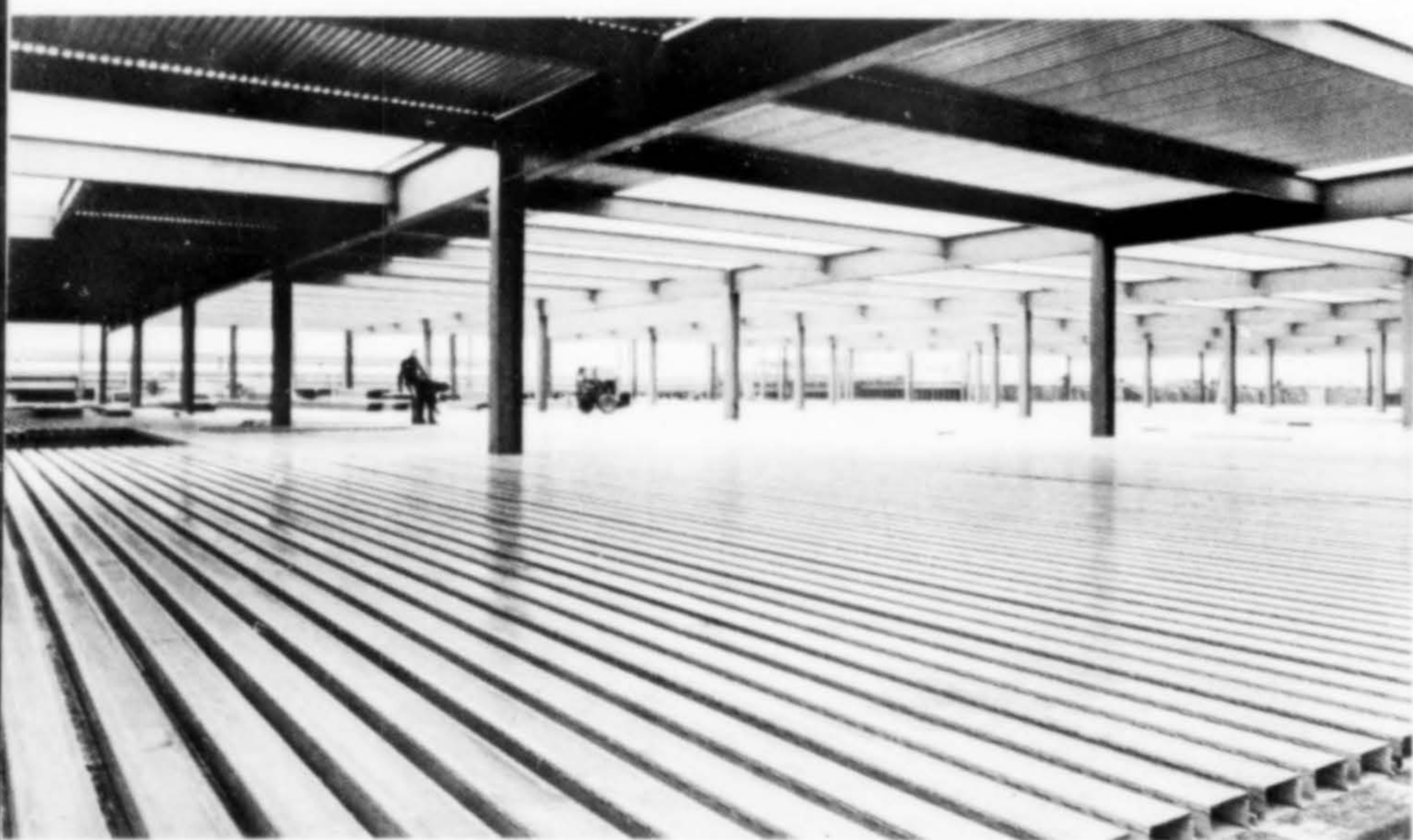
Typical Q-Lock ® Floor installation.
