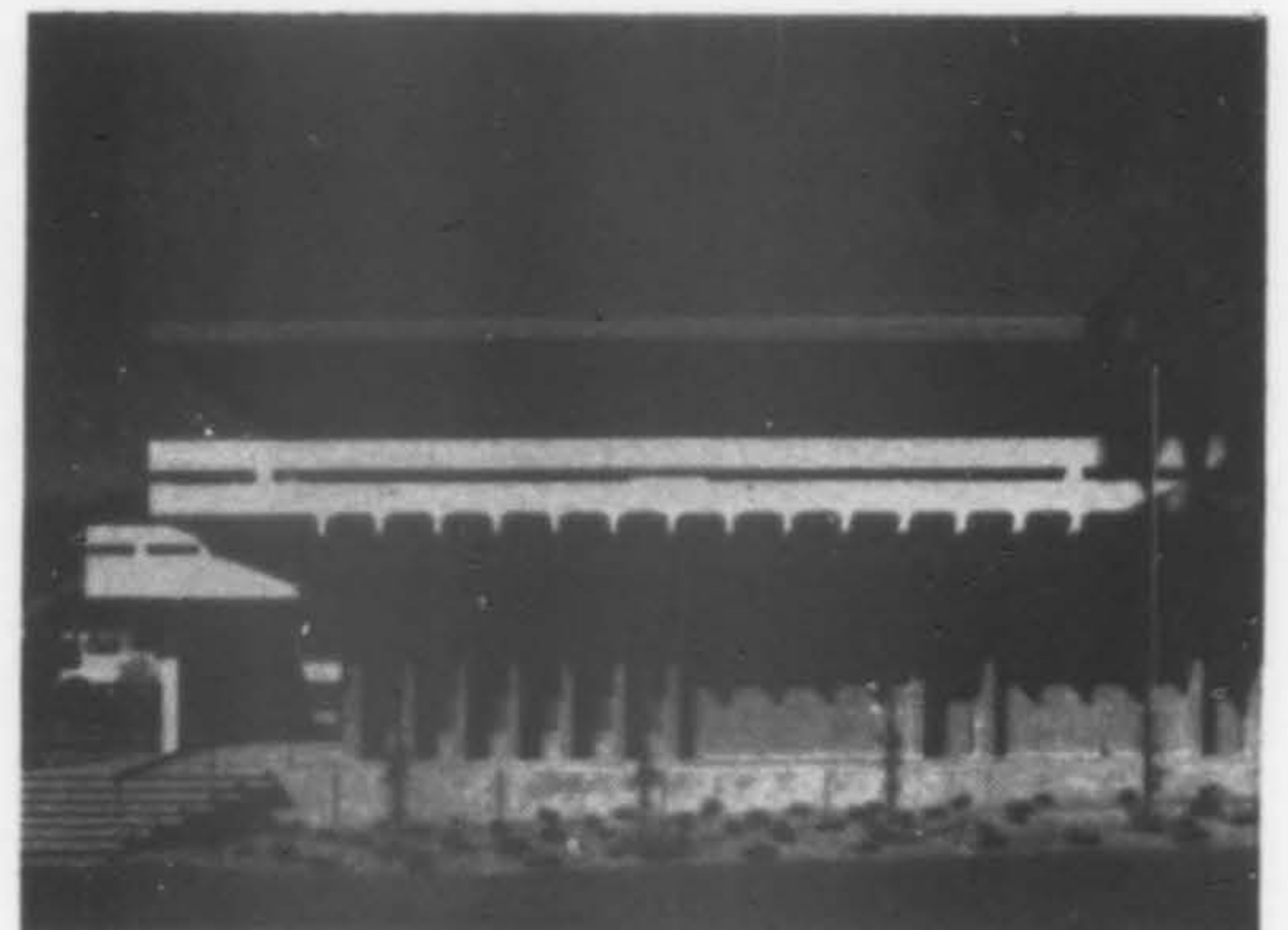
PHYSICAL SCIENCE BUILDING, Citrus College. Merit Award. Neptune & Thomas, architects.
