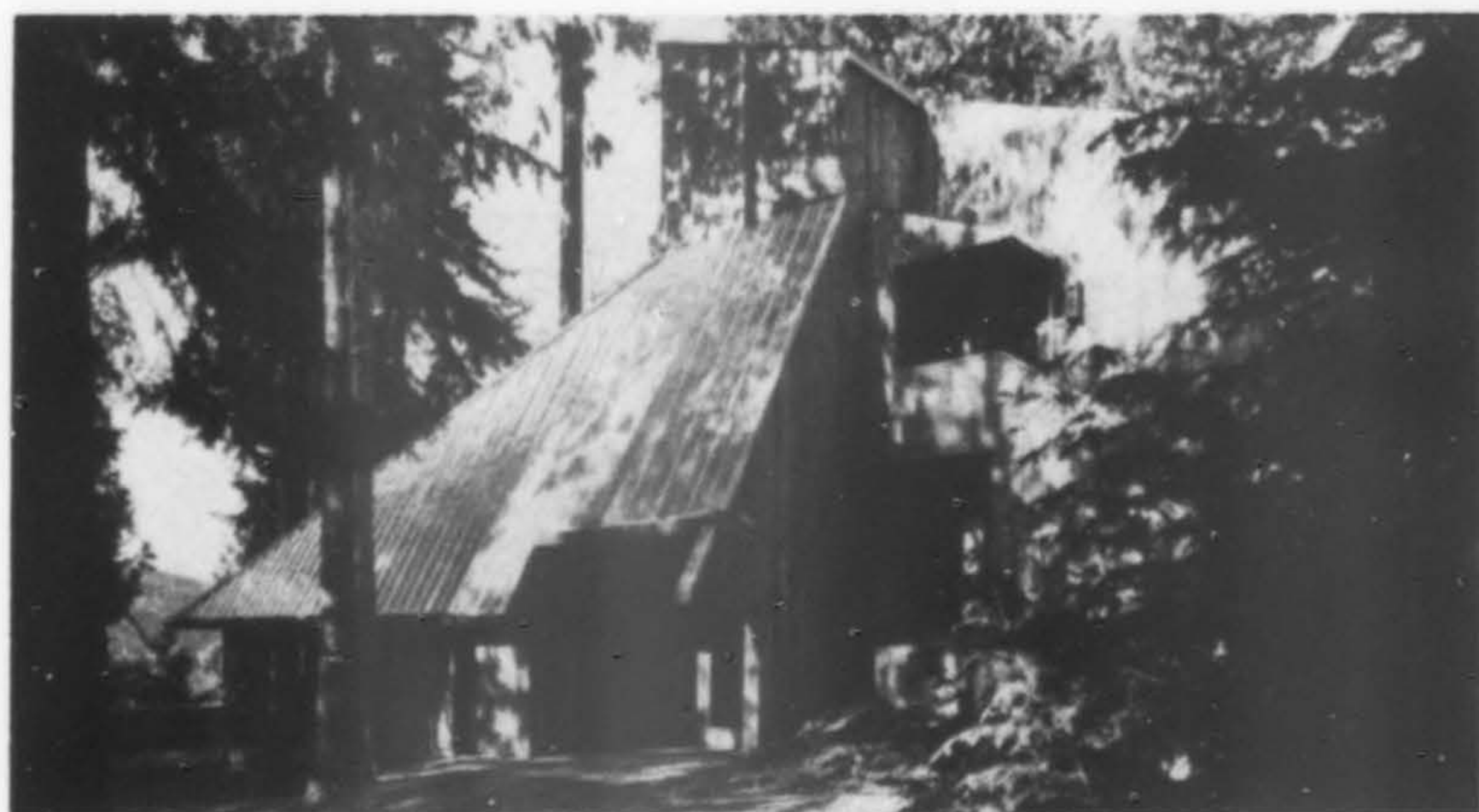
CAMP BROTHERHOOD Dormitory, Mount Vernon. Award of Merit. Robert Small and Environ '68, architect.
