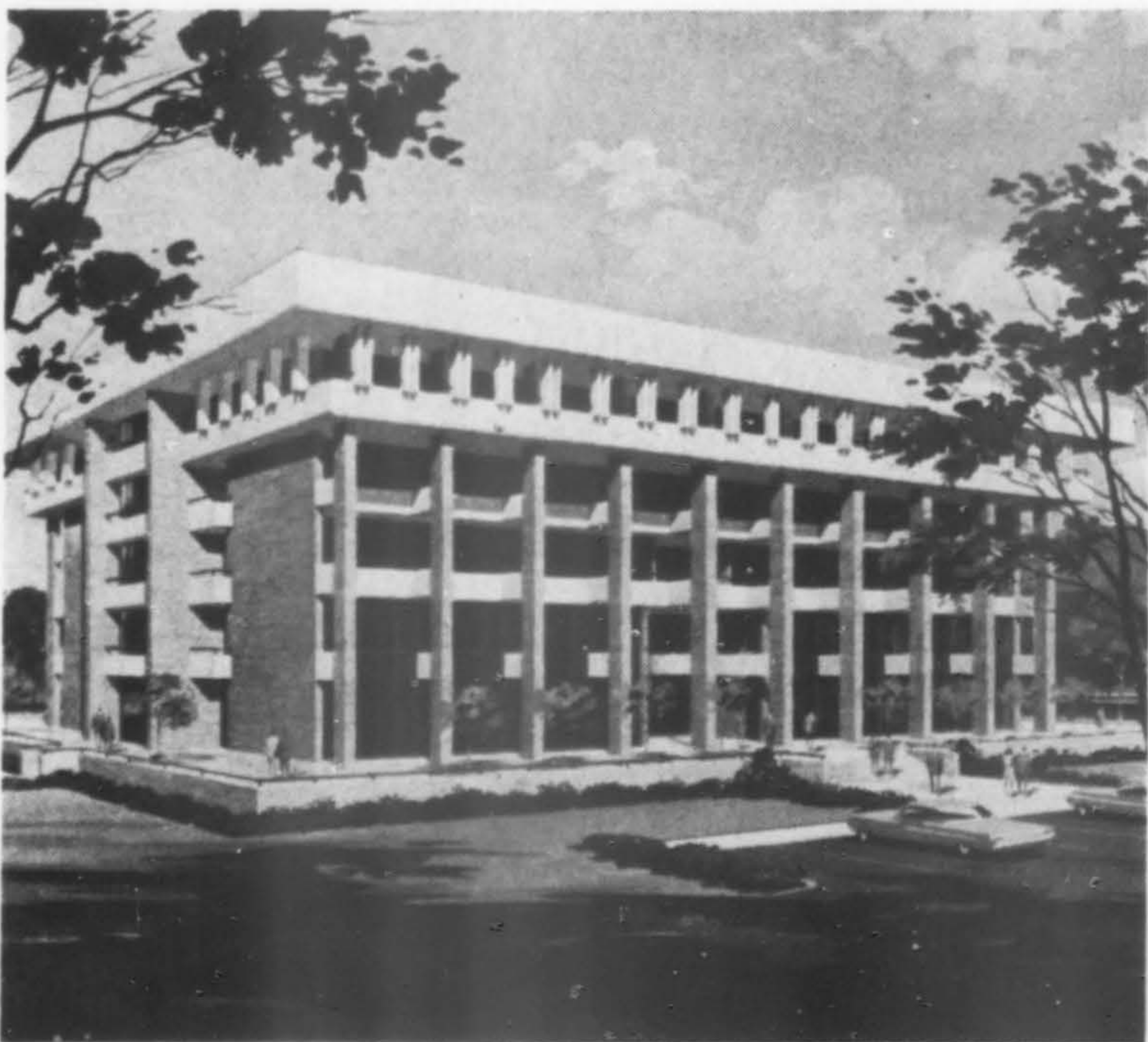
HEADQUARTERS OFFICE BUILDING for Morrison-Knudsen Co., Inc., Boise, Idaho, will be five stories with a full basement and provision for an additional two stories as needed. The new building, occupying an eight-acre site, will rise from a raised plaza with a four-story inner court. The building will be basically a reinforced concrete structure with vertical exterior columns faced with gray brick. Architect: Wayland, Cline & Smull.
