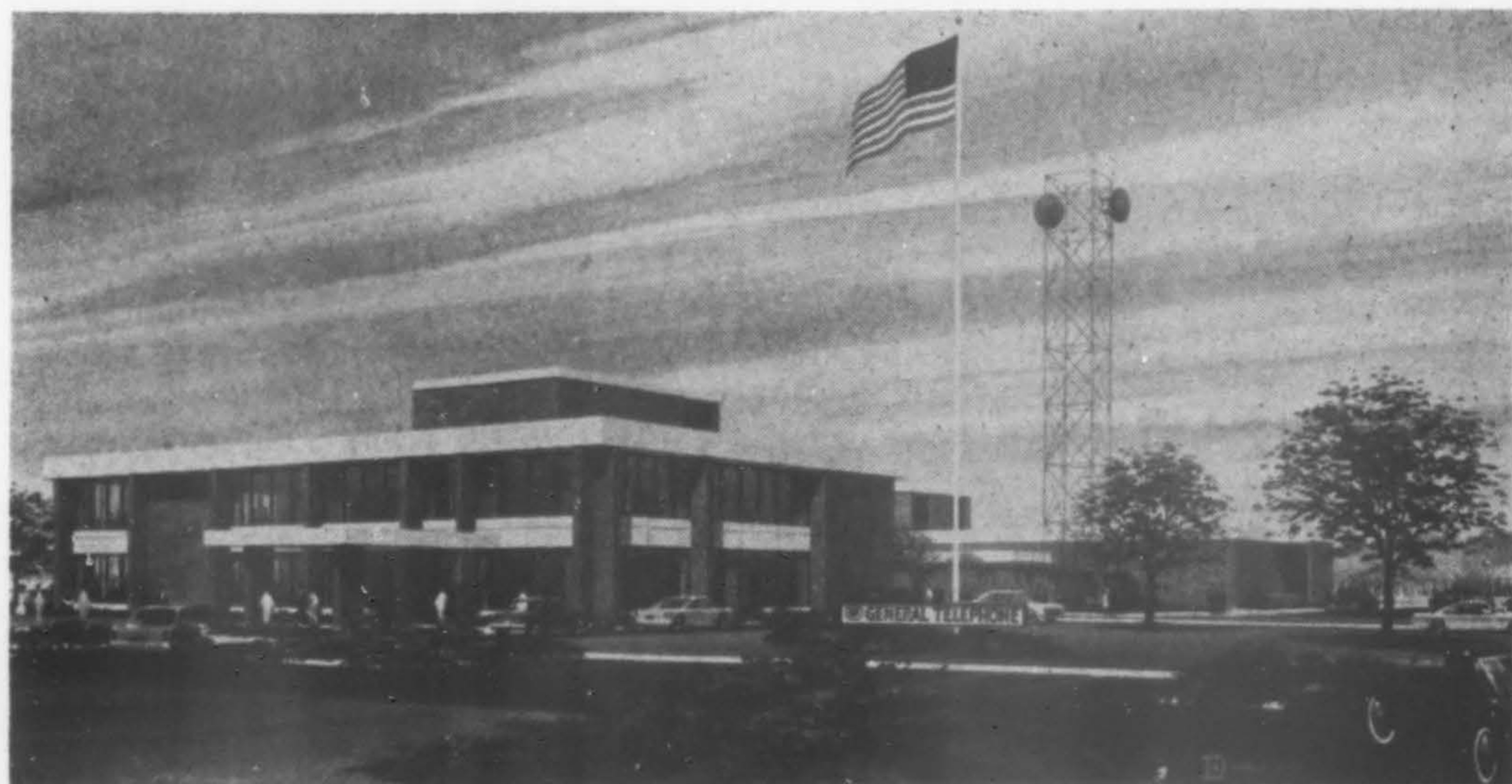
TOLL CENTER and District Office , General Telephone Company, Coeur d'Alene, Idaho, is two stories, concrete with brick veneer structure. The complex includes a cafeteria linking the two buildings with a landscaped courtyard. Cost: $1.5 million (52,000 sq. ft.). Architect: Decker, Kolb & Stansfield.
