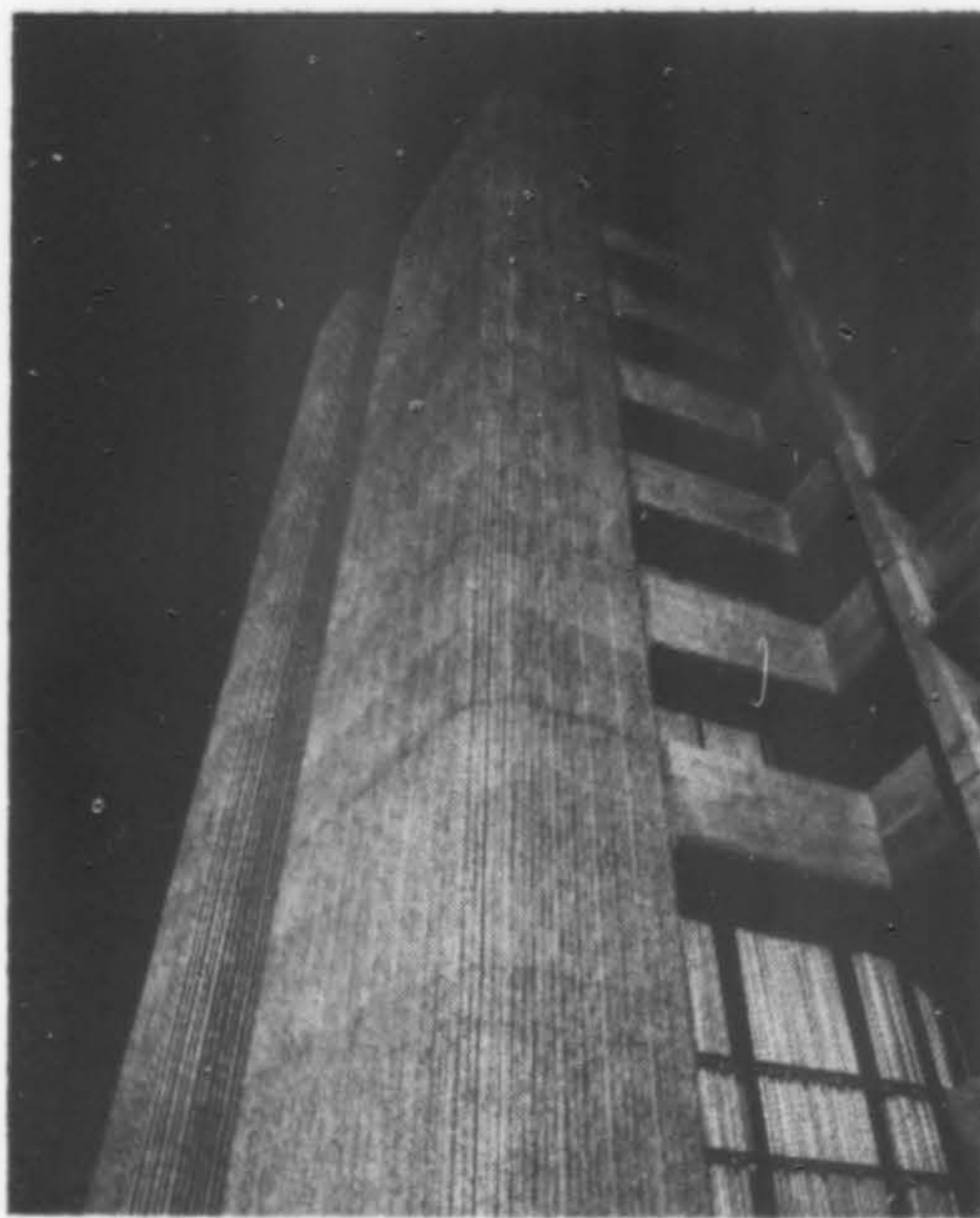
LIBERTY BUILDING, Los Angeles, Kurt Meyer & Associates, architects.
