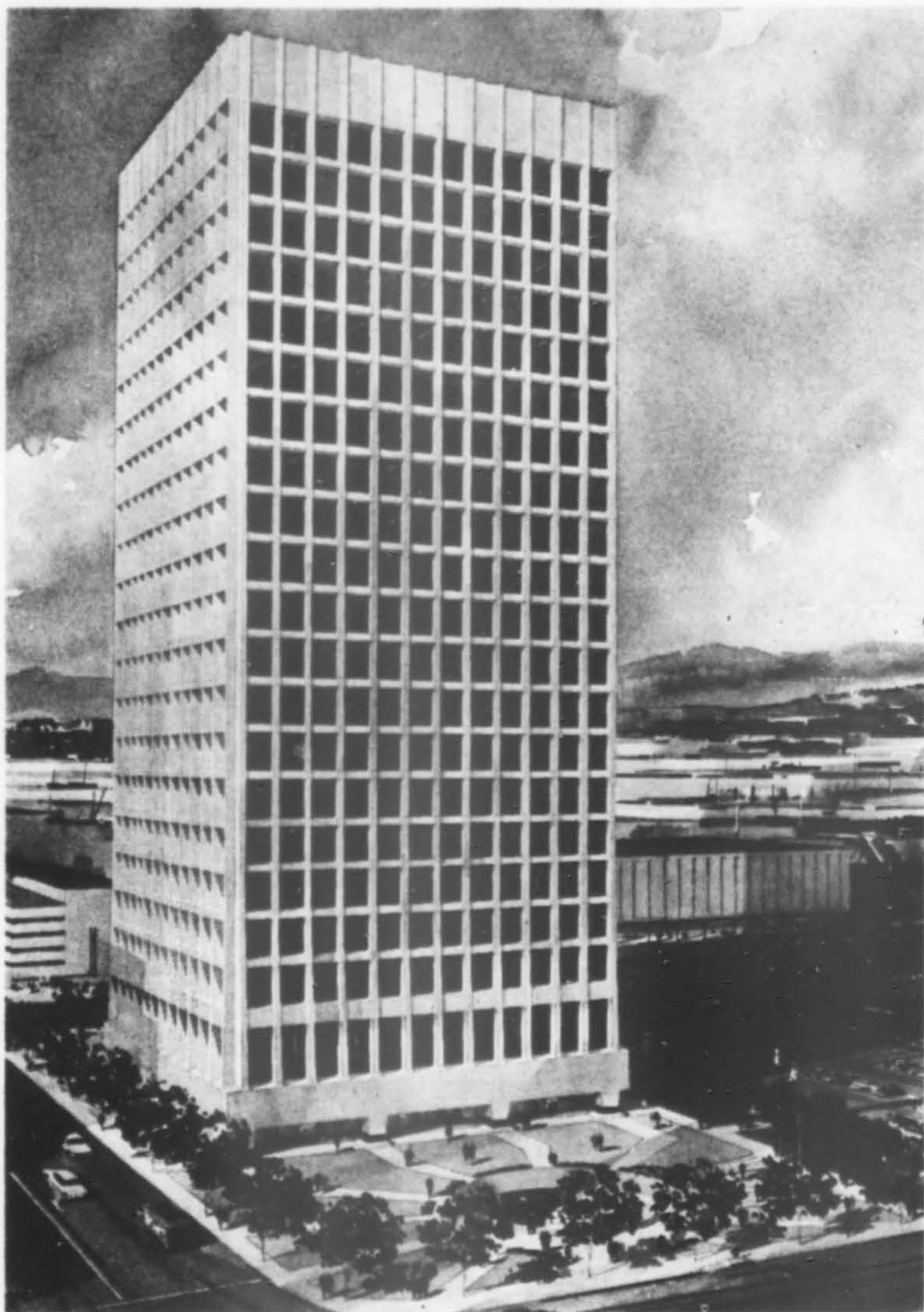
BANK OF WASHINGTON PLAZA , Tacoma, Washington, will occupy a full block. The 22-story building will be a concrete structure with recessed tinted glass windows. Cost: $12 million. Architects: Skidmore, Owings & Merrill; Lea, Pearson & Richards, associate architects.
