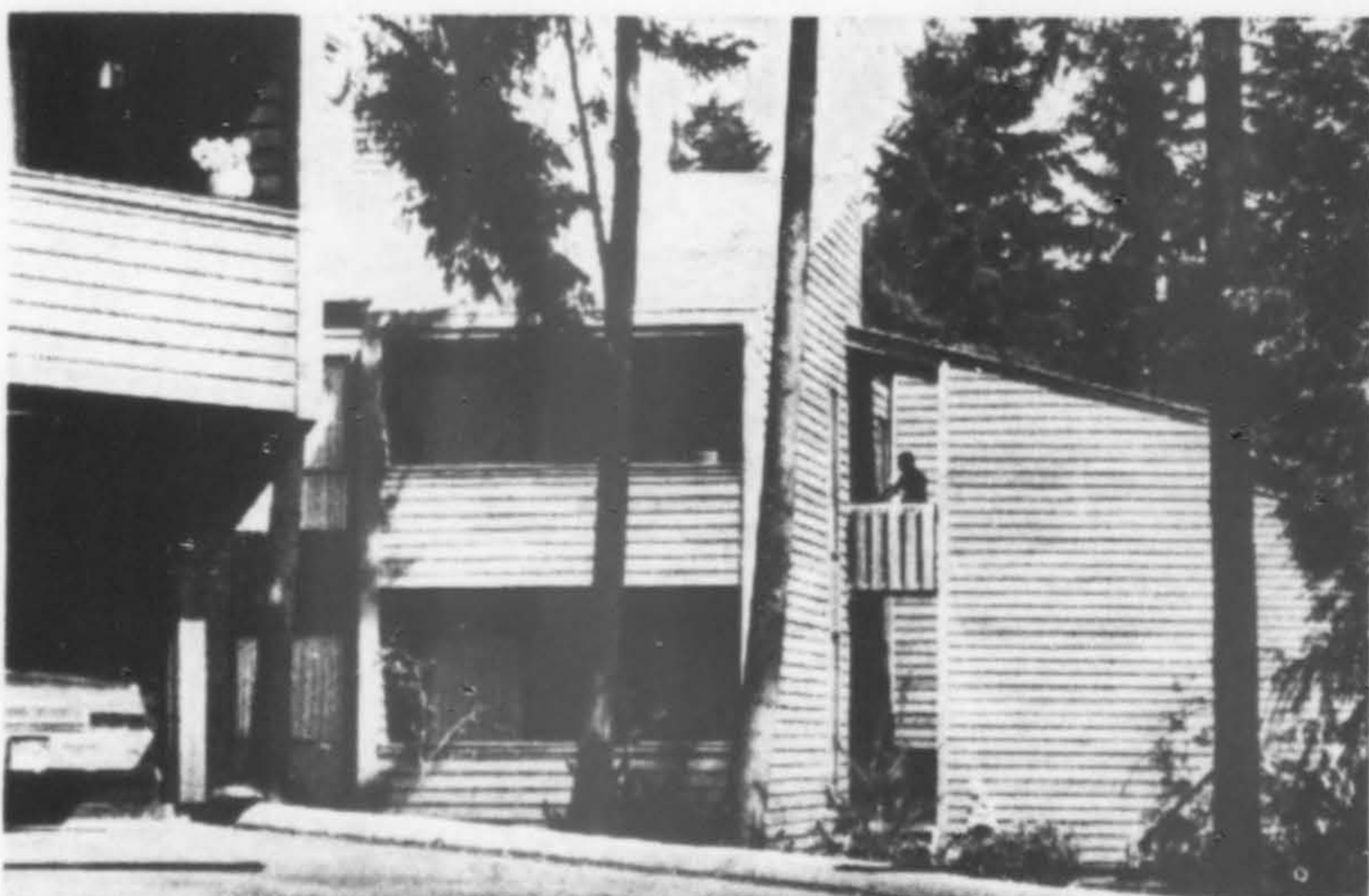
LAKERIDGE VIEW APARTMENTS, Bellevue, Washington. Commendation Award. Zaik/Miller, architects.
