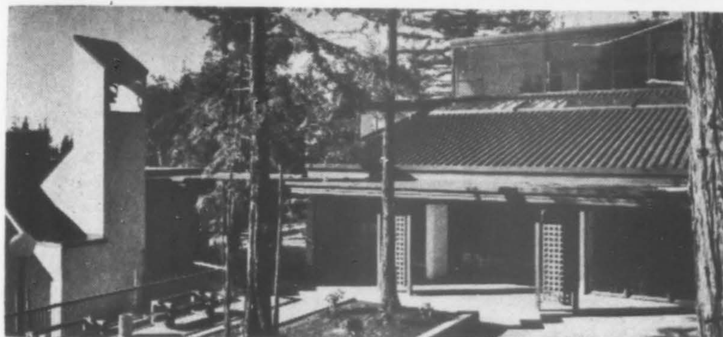
MERRILL COLLEGE , University of California, Santa Cruz. Award of Merit. Worley K. Wong, architect; John C. Campbell, A.I.D.
