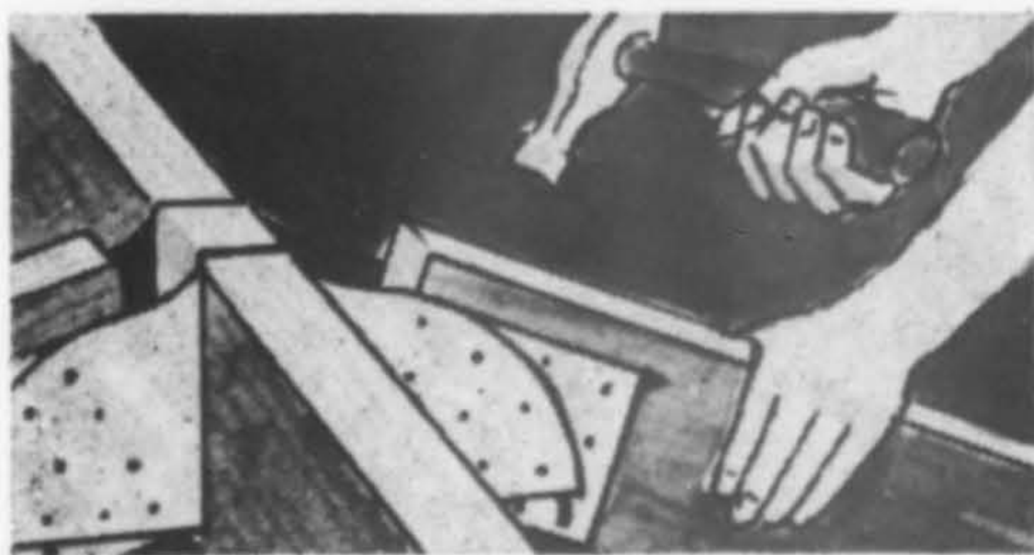
ADJUST TO PITCH, NAIL INTO POSITION EASILY
