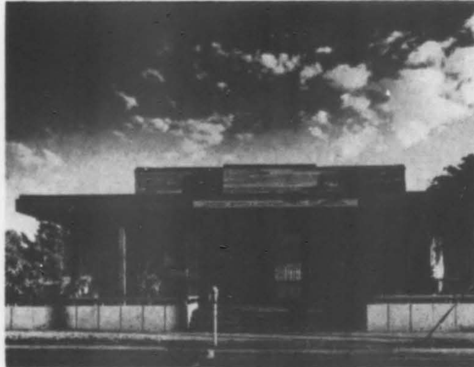
U. S. NATIONAL BANK, Eugene. Merit Award. Wilmsen, Endicott, Green & Associates, architects.
