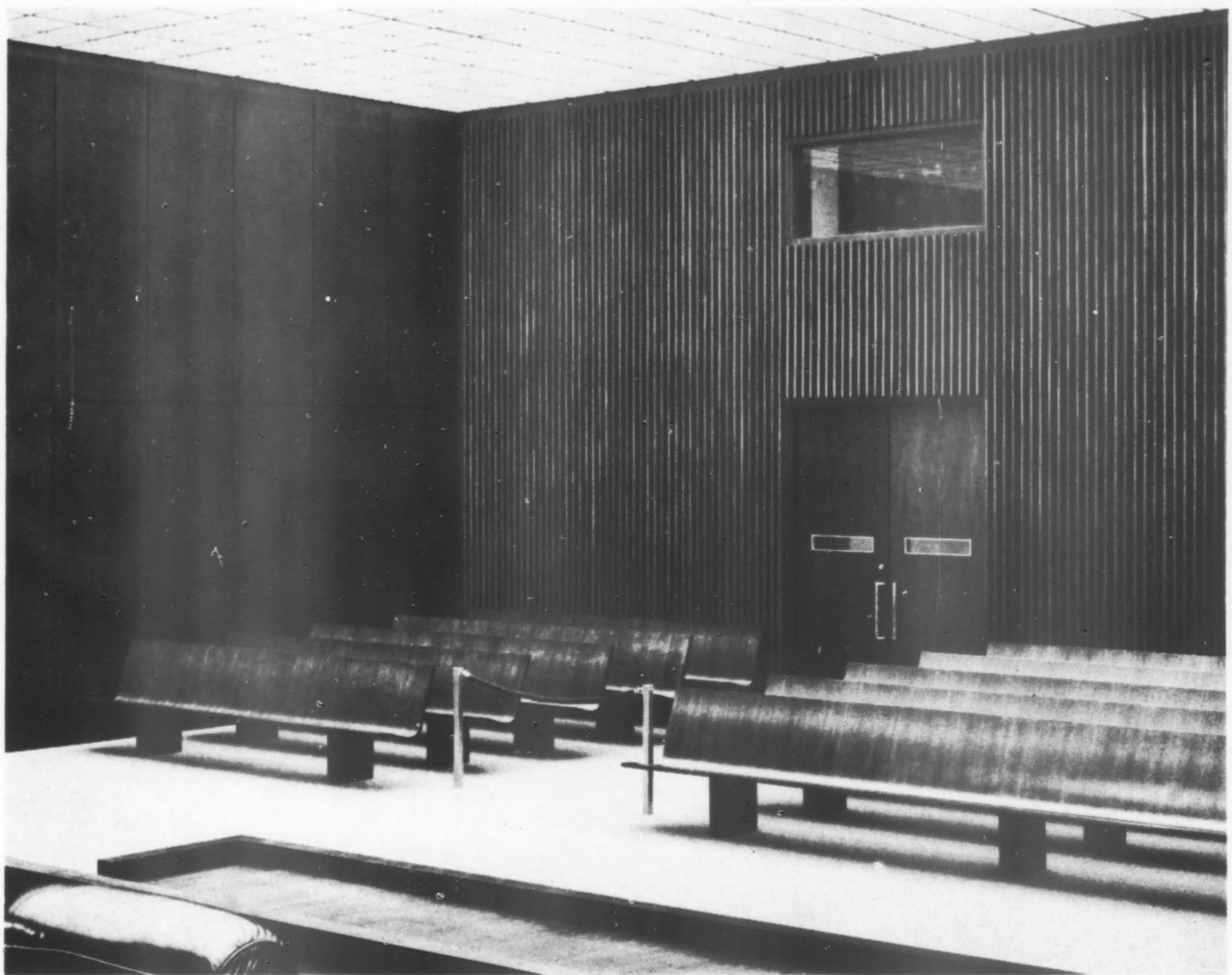
Weyerhaeuser Blueprint matched prefinished walnut paneling and doors
