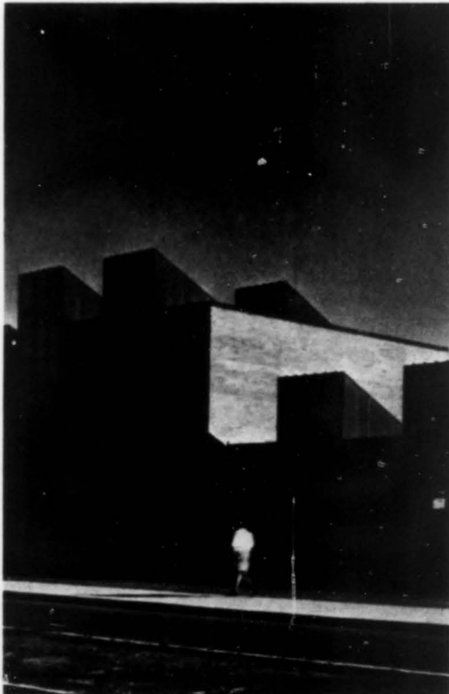
FINE and APPLIED ARTS Building, Central Washington State College, Ellensburg. Merit Award. Kirk, Wallace, McKinley & Associates, architects.
