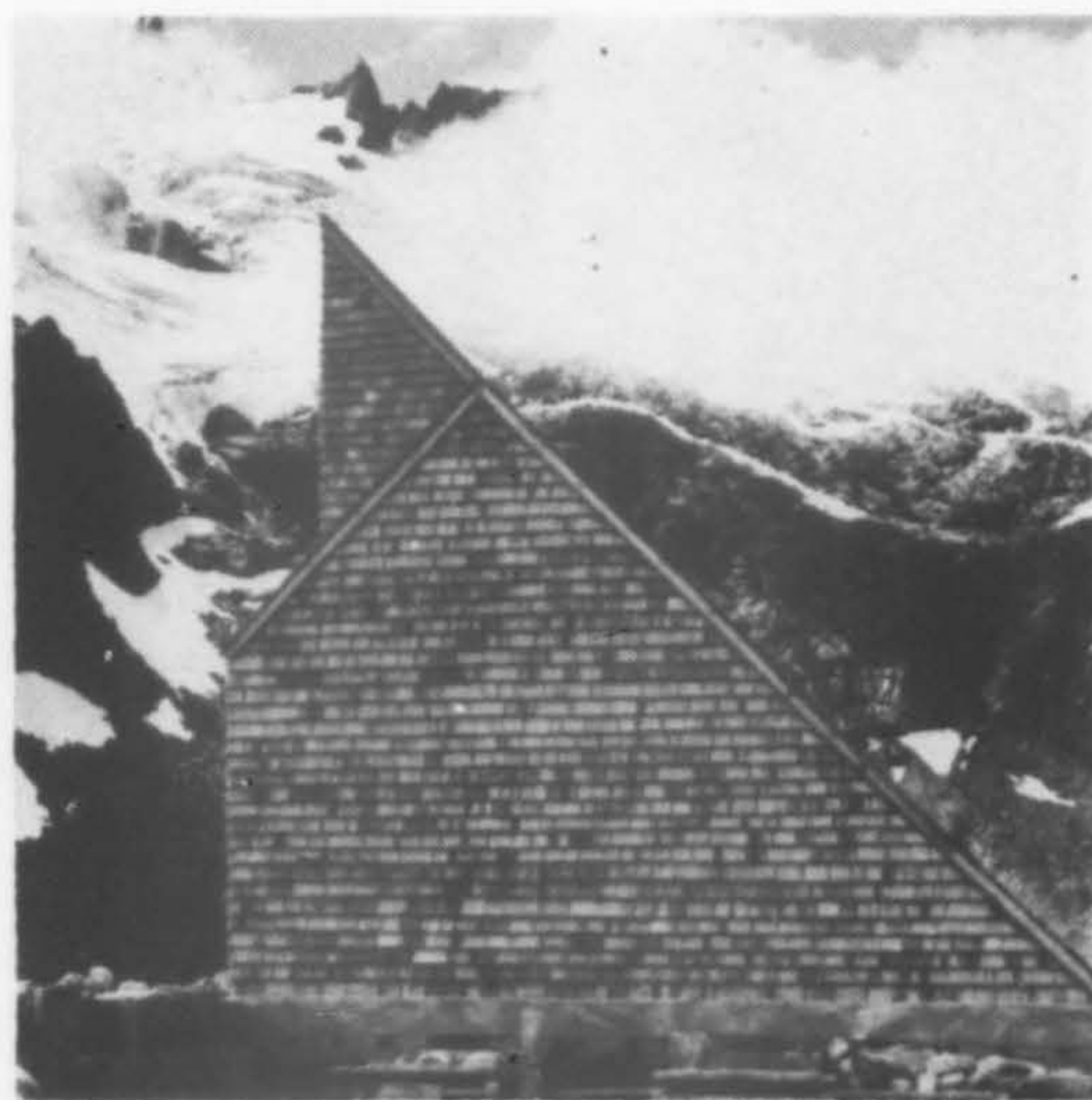
GLACIER GAUGING Station , South Cascades. Merit Award. Harris, Reed & Litzenberger, architect.
