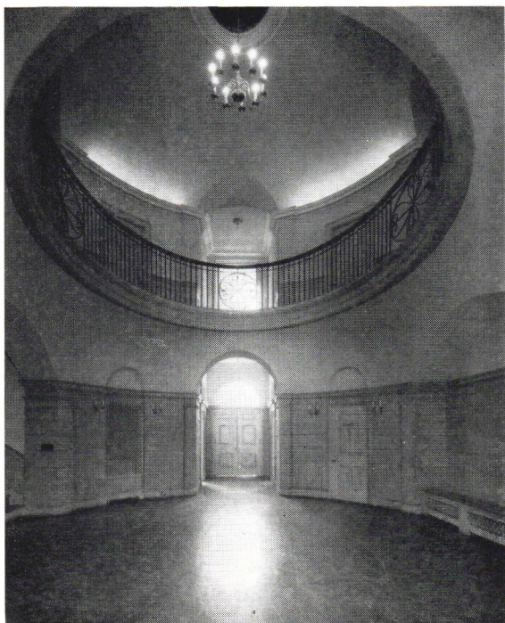
Rotunda, Administration Building
