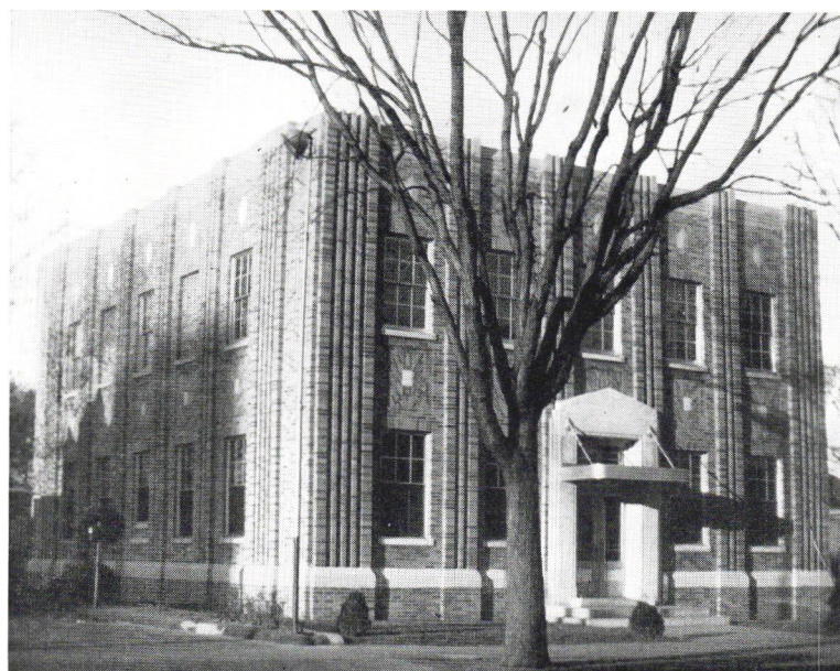
CENTRAL OFFICE BUILDING CAROLINA TELEPHONE & TELEGRAPH CO. Wilson, North Carolina
