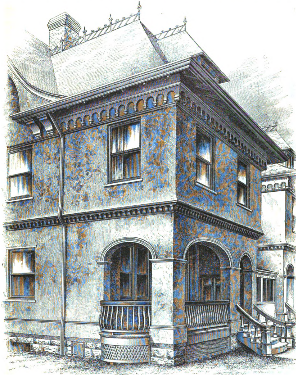
Metal Lath and Cement Construction.—General View of Building at one of the Front Corners.
