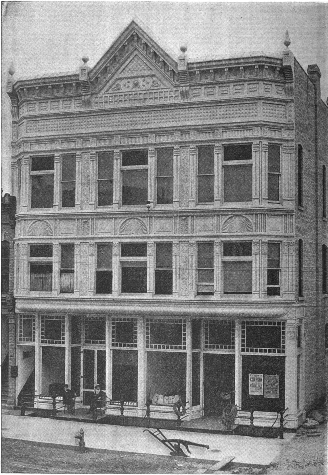
An Indiana Business Building.—General View Reproduced from Photograph.—O. H. Dirham, Architect, South Bend, Ind.
