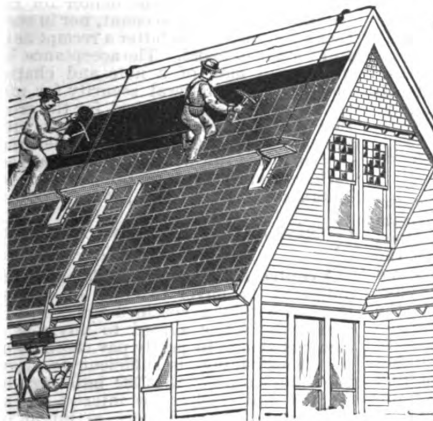
Fig. 15.—Showing Application of Slaters' Scaffold Bracket.
