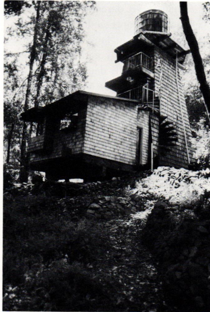
THREE-STORY WATER TOWER COTTAGE.
