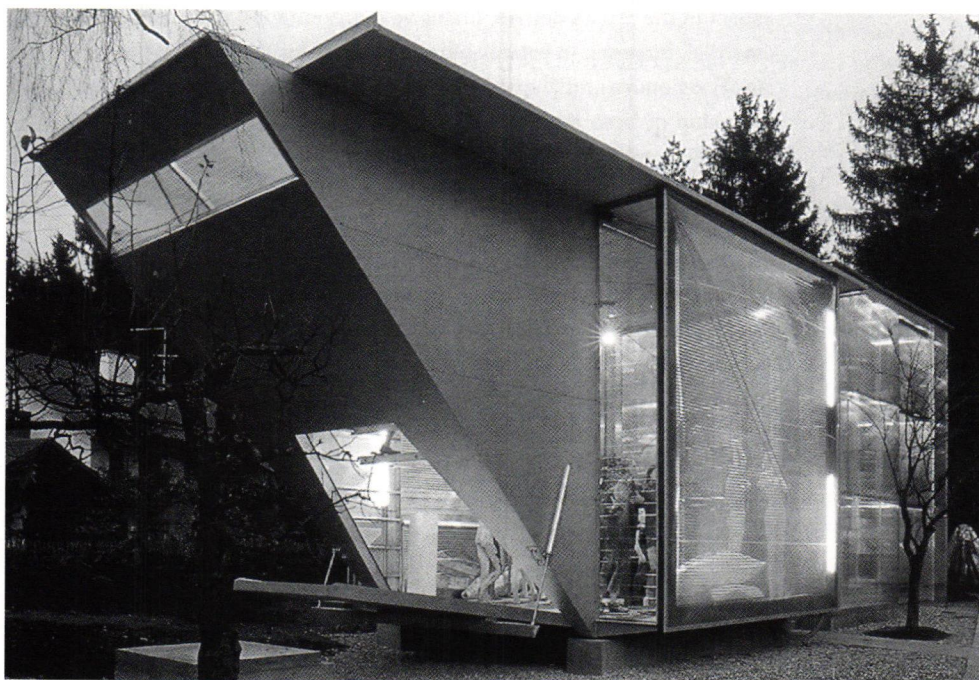
The Atelier Mimesis, 1993, located near Munich, Germany, was constructed as a work studio and adjoining exhibition space for sculptor Beate Schubert by the architectural team of Peter Haimerl, Ralph Feldmeier, and Maria Laurent. The flexible building design incorporates scaffolding, aluminum plates, Plexiglas sheeting, and air-inflated Teflon foliate. (from Towards a New Museum )
