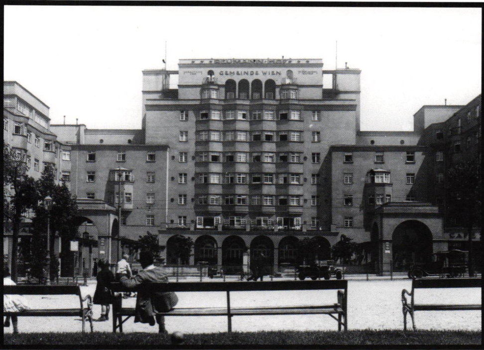
Designed by Hubert Gessner, the Reumannhof was completed in 1924. The project, containing 485 apartments, 22 stores, and a child-care center, was one of the largest of the Vienna Gemeindebauten .
