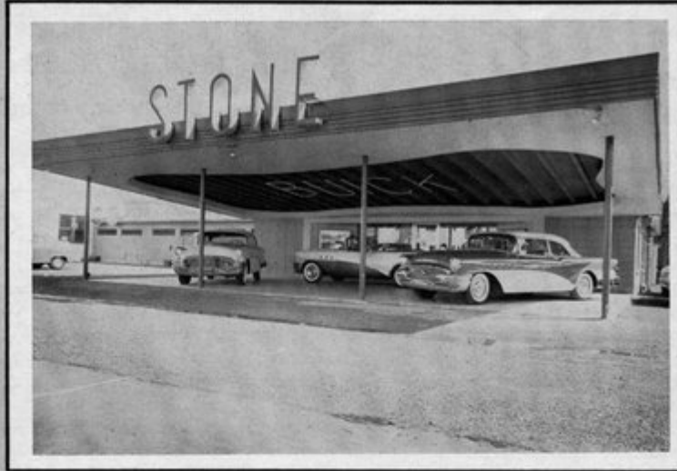
The new Stone Buick Building in Fort Pierce . . . Kendall P. Starratt, Architect . . . Mistik & Lester, General Contractor . . . "Double Tee" Prestressed Concrete Roof for building and open show room supplied by R. H. Wright & Son, Inc., Fort Lauderdale.
