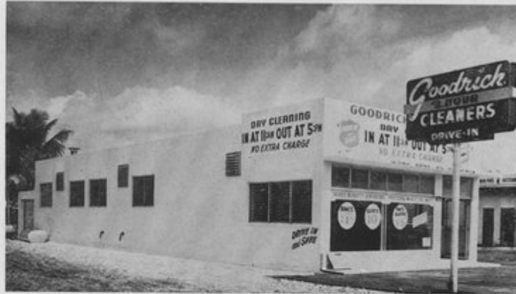
New Goodrich Building in Hialeah built with JALOCRETE Security Windows.
