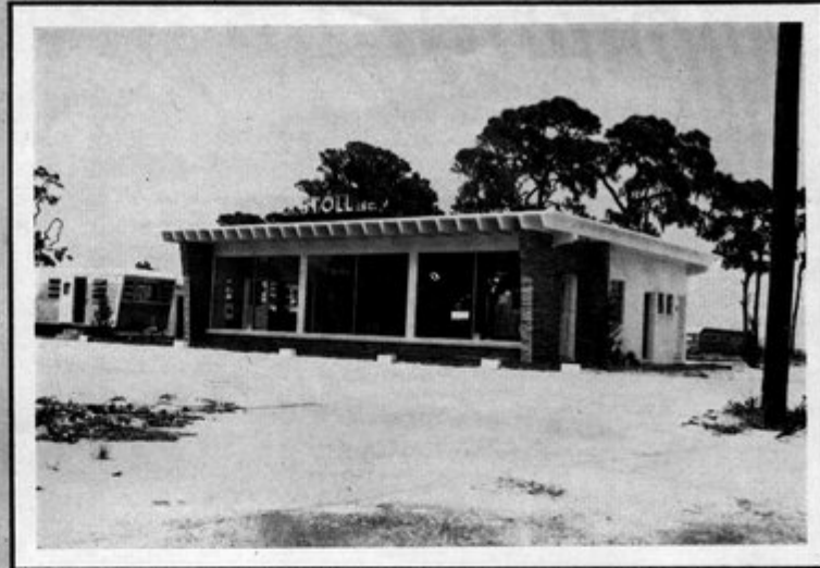
Office and Display Room of C. J. Stoll Inc., at Sarasota . . . Elden Ray, Contractor . . . Kannenberg & Hanebuth, Architects . . . Double Tee prestressed roof deck supplied by West Coast Shell Corp., Sarasota.
