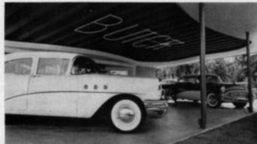
Outdoor showroom of Stone Buick agency, Ft. Pierce, Fla., showing combination of LEAP exposed double tees and lighted cove in modernistic design.
