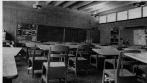
Interior of classroom at the Stuart, Fla., elementary school showing effect obtained through the use of exposed LEAP Double Tees.
