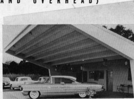
Outdoor showroom of Lincoln-Mercury dealer at Bartow, Florida, showing modernistic effect of LEAP Prestressed Concrete.
