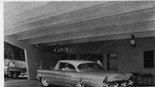
LEAP Tees are left exposed, then painted for pleasing effect. This type of roof is strong, adds beauty and requires no upkeep.
