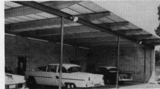
Service department of Lincoln-Mercury dealer at Bartow, demonstrates versatility of LEAP Prestressed Concrete products for all types of building.
