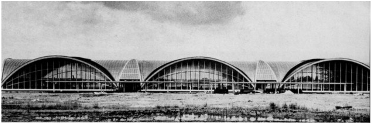
Above, the St. Louis Municipal Airport Terminal Building, one of the five First Honor Awards, for which the firm of Hellmuth, Yamasaki and Lienweber, St. Louis and Detroit, were the architects.
