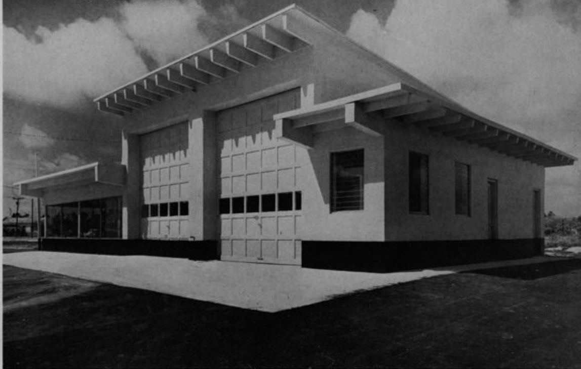
Service Station for Superior Oil Co. Twin-T units in eight-inch, twelve-inch and fourteen-inch depths were selected for the roof structure as required by the various spans.
