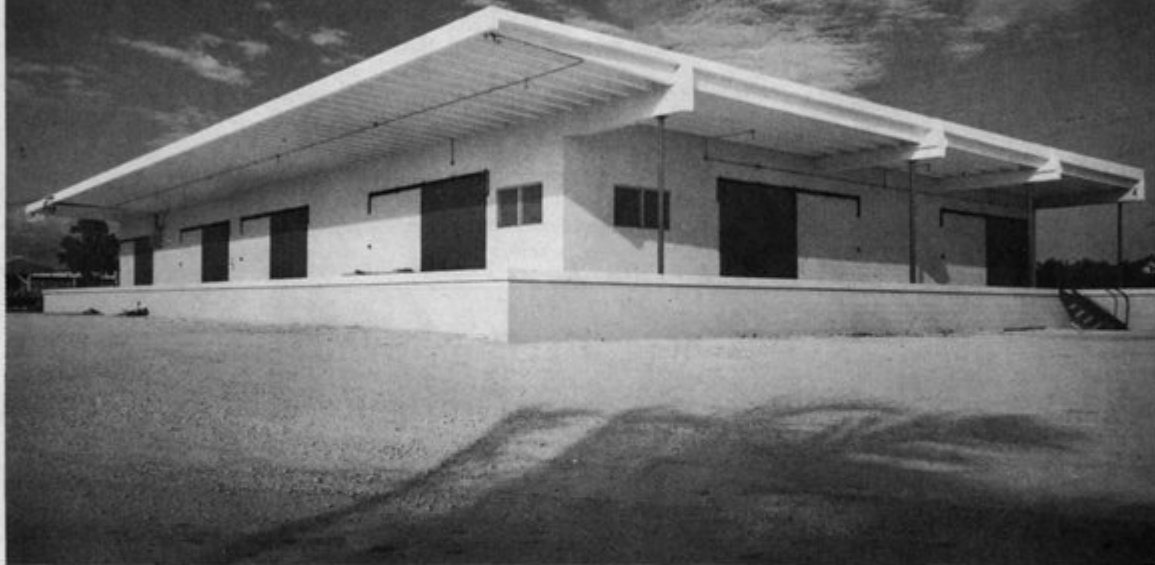
Warehouse building for H. L. Cox & Son, Princeton, Florida. Harry E. Penney, architect; Linton Connor, general contractor. Hollostone pre-cast structural beams and Twin T roof panels provide a 15-foot cantilever over loading dock.
