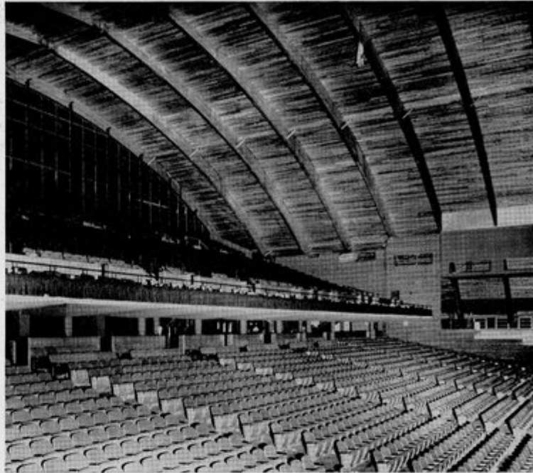
This interior view of the West Palm Beach Jai-Alai Fronton indicates the scale of the huge glue laminated segmental arches which are low-buttressed at the base and hinged at the crown. Arches are spaced 16 feet on centers, are braced by two series of horizontal purlins on each side and are roofed with solid 4 by 5-inch wood decking of western red cedar. Arches themselves are laminated with Southern pine.
