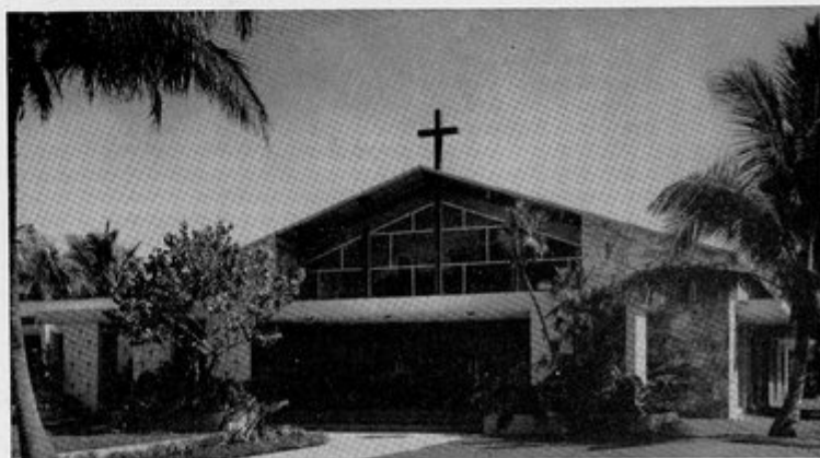
On the exterior of the Church of the Resurrection, arch framing and roof construction have been exposed as integral parts of the building design — a practical matter since the glued laminated units usually require no unsightly mechanical connectors for efficient use.
