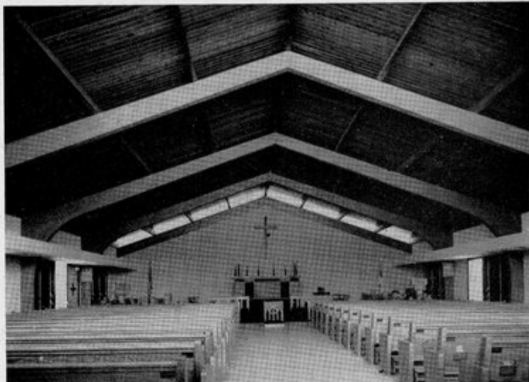
Typical of the use of glued laminated arches for church or meeting hall roofs is the interior of the Church of the Resurrection at Biscayne Park, for which Robert K. Frese, Miami, was architect.
