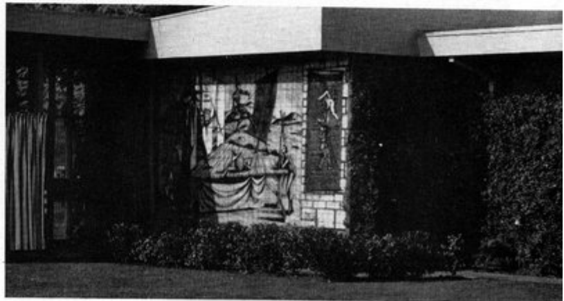
Colorful glass tile has been used in decorative panels on this Beverly Hills, Cal., house. Photo from a book by E. Bitterman, courtesy of Reinhold Corp.
