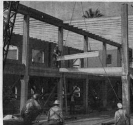
Large photo, completed building. Above: Placing a roof girder. Below: Placing a precast floor joist. Alec Arany, engineer, John K. Minasian, consulting structural engineer, J. A. McNeil Company, Inc., contractor, all of Los Angeles.
