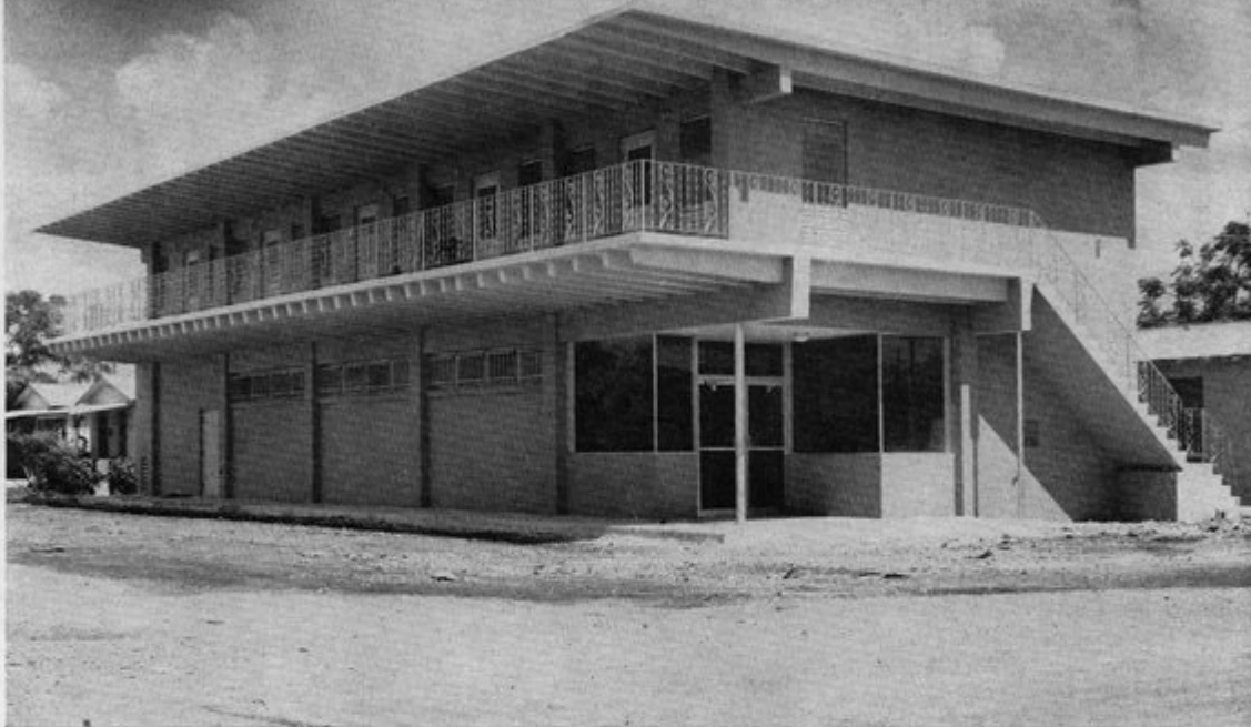
Store and apartment building, for which Henry E. Brown, Jr., was the architect, utilizes Hollostone pre-cast stairs and Hollostone Twin T units, the latter forming a 9-foot cantilever balcony and roof overhang.
