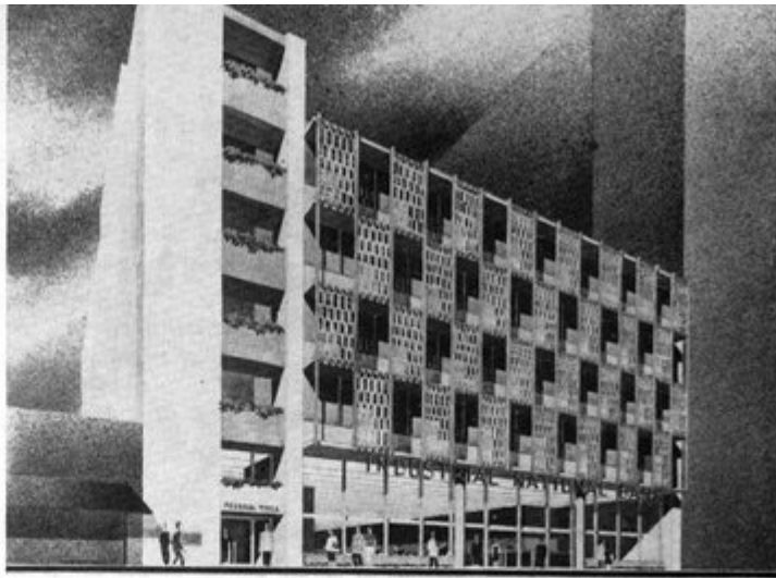
Decorative grilles on the facade of Miami's Industrial National Bank, by Edwin T. Reeder Associates, will be of gold-anodized aluminum. Machine-fabricated from an original design, they offer another example of how a single motif can be adapted to a multiplicity of panels.
