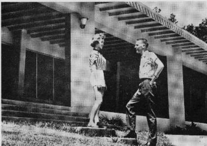
Roofed with prestressed double-T slabs, this new dormitory for women at Florida Southern College, Lakeland, C. Dale Dykema, architect, indicates that prestressed units can be easily designed to residential scale as well as to the larger spans required by the heavier loadings and operating conditions of industrial and commercial structures.
