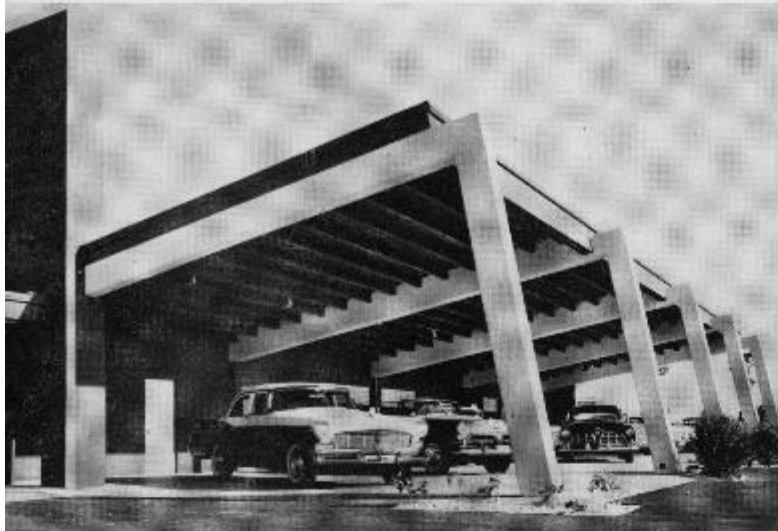
Another all-prestressed building, an auto-agency building at Pompano Beach for which Cranford Sproul was the architect. Open-air display terrace is roofed with double-T units supported by prestressed beams which are anchored to inclined columns.
