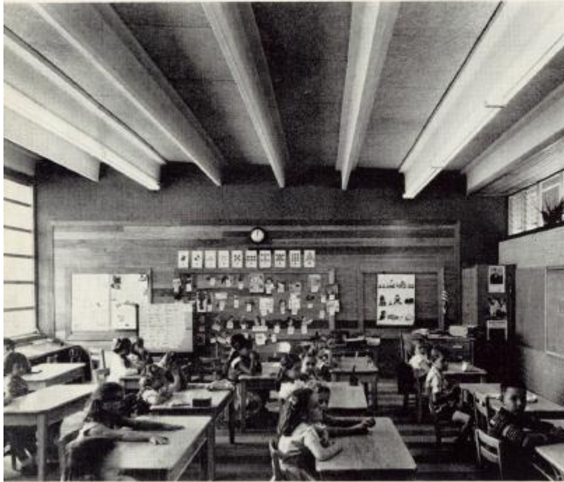
Extensive use of prestressed units has been made in the Elementary School at Stuart, Starratt and Armstrong, architects. Classrooms, above, are roofed with insulating structural slabs, keyed in, and grouted to T-beams. Beams bear on job-poured longitudinal beams which are cantilevered to provide bearings for double-T slabs forming a canopy over a walkway, top.
