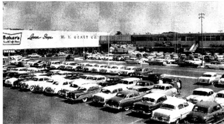
In Miami's 79th Street Shopping Center, for which Robert Fitch Smith was architect, the need for adequate parking directly influenced the building design. Note bridge over driveway connecting parking lots and the outdoor stairway which serves second-floor offices directly from parking area.
