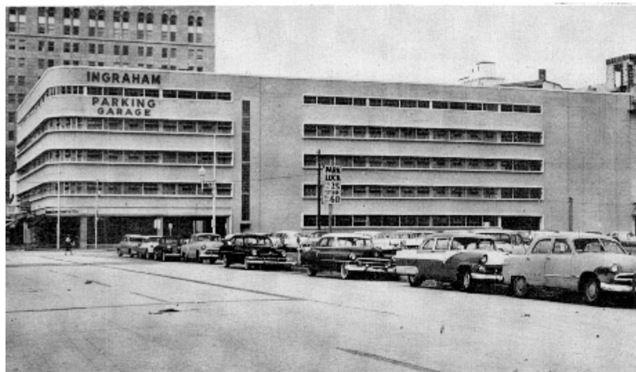
Experience has shown provision of adequate parking facilities in central business districts tends to maintain, even increase, property values. This is one of several ramp garages in downtown Miami. It has a rated capacity of 539 cars, was built in 1949. Robert Law Weed & Associates were the architects.
