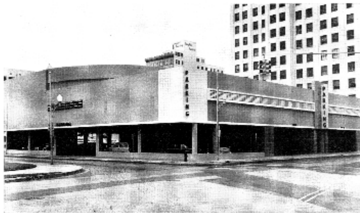
Newest of Miami's parking garages is this structure opened last summer in the heart of the central business district. Designed by Stephan Zachar, architect, it has a rated capacity of 274 cars, is planned for more floors.
