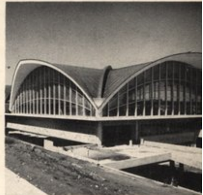
Airport Building, St. Louis, Mo., employs intersecting shells, 4½-inches thick throughout. Architects were Hellmuth, Yamasaki and Leinweber; the structural engineer, William G. Becker.
