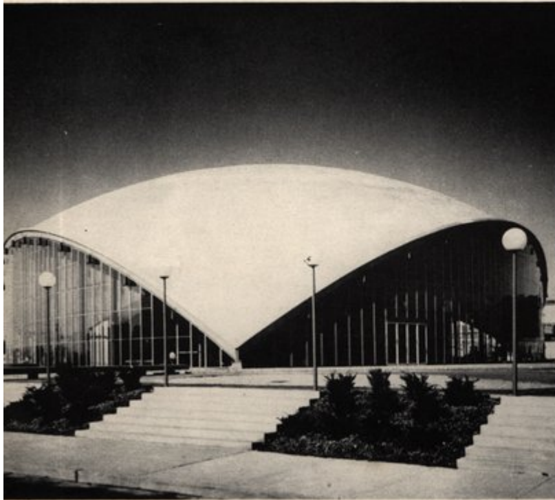
The thin-shell covering of the Kresge Auditorium for Massachusetts Institute of Technology at Cambridge, Mass. has ground support at only three points which are about 175 feet apart. Cost of the dome was about 10 percent of the building. Architect was Eero Saarinen, FAIA; consulting engineers, Amman and Whitney.
