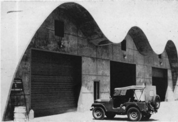
Top, gymnasium roof shell, supported by end columns, seems to float. Eberle Smith, Detroit, architect. Above, roof of armory building in Oklahoma, Paul Harris, architect, suggests the varied shapes possible; and armory dome below shows possibility of piercing for vents or skylights.
