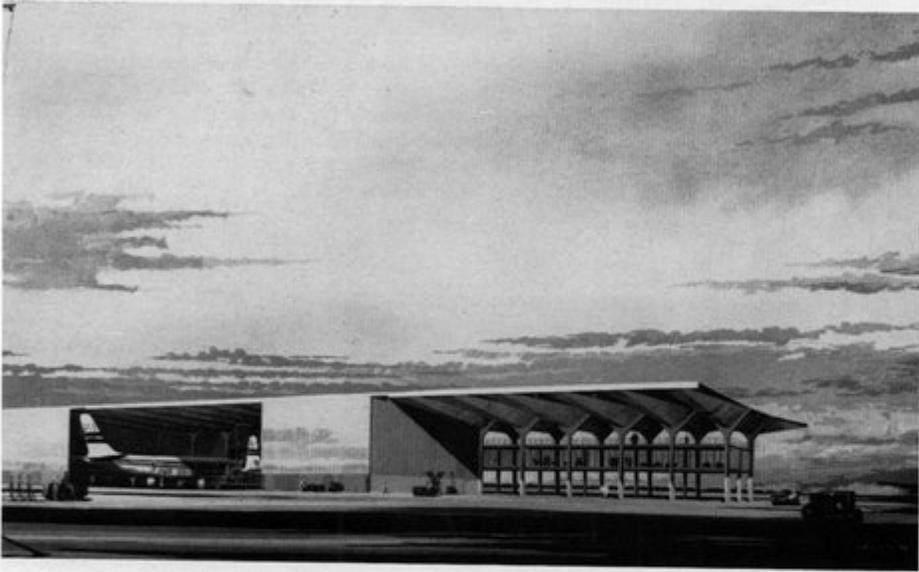
Measuring 20 by 34 inches in the original, this rendering shows the maintenance hangar for National Airlines as designed with a folded plate concrete structure by Weed, Russell, Johnson, Associates. The building is now in process of construction.
