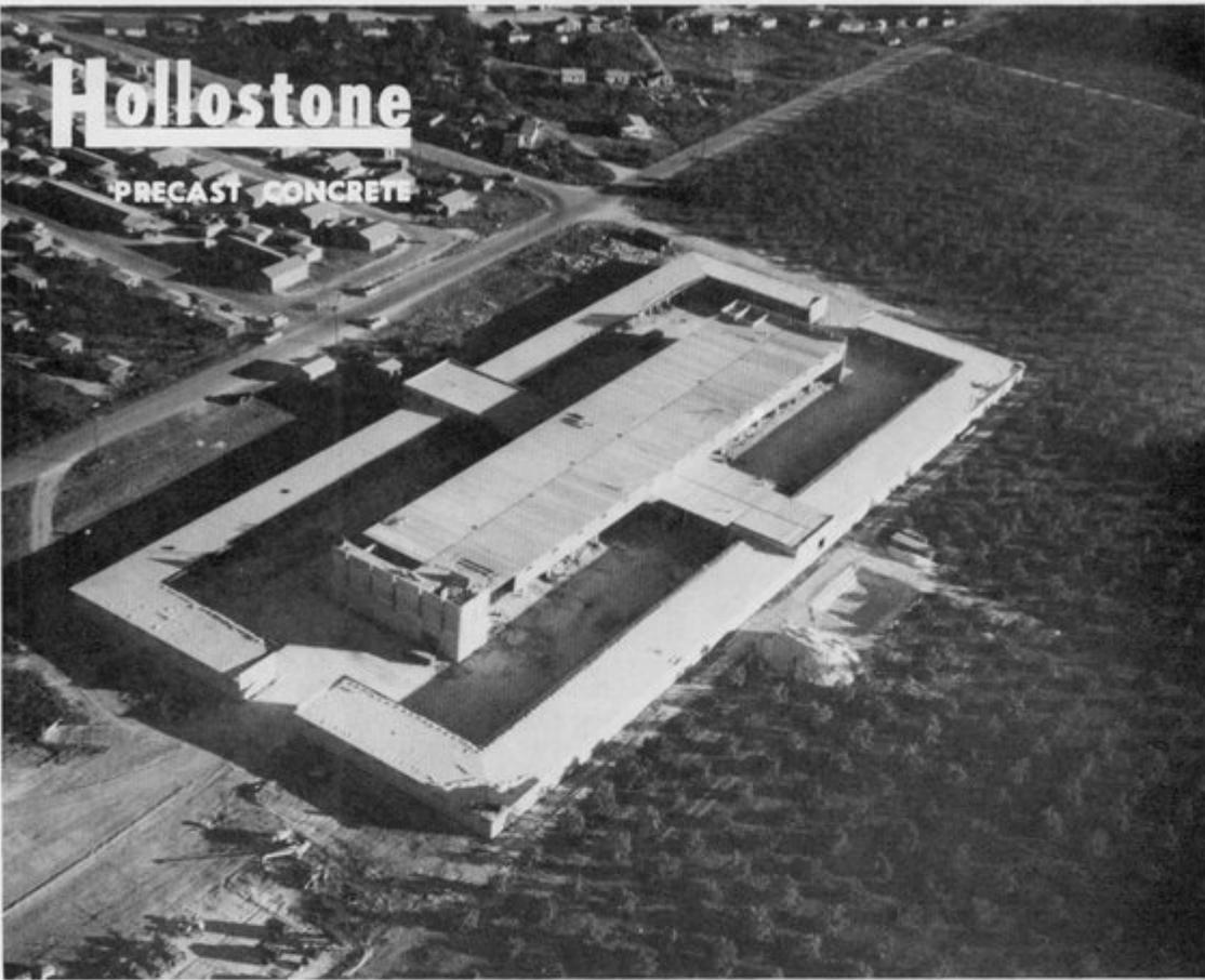
Throughout this five-acre industrial building for the B & L Farms Co. Hollostone precast units have been used as integral parts of the construction. These include one-and two-story columns, beams, wall panels and floor and roof units.
