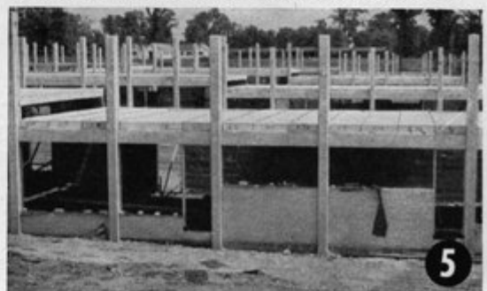
4 General view before roof spandrel beams and roof slabs were erected.
