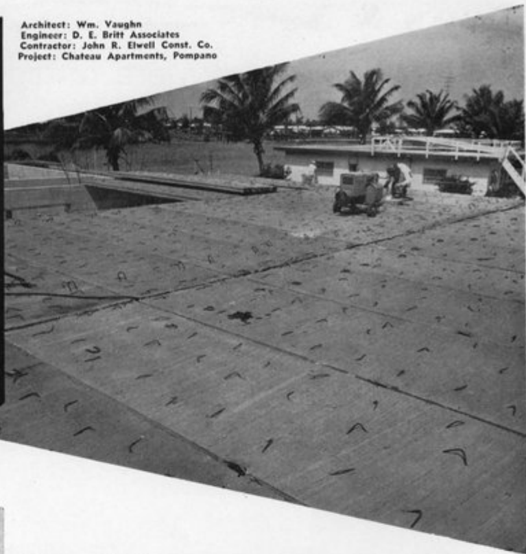
Slabs are cast in all-steel forms for uniformity. Mass production technique assures availability for on-time delivery. Modular 4" width, spans up to 26'.
