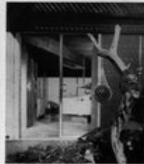
CHERFUL KITCHEN has wall of floor to ceiling fixed glass at one end, and 2' Ador sliding glass door at other end.
