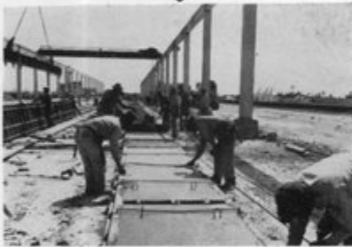
Slabs are cast in all-steel forms for uniformity. Mass production technique assures availability for on-time delivery. Modular 4" width, spans up to 26'.
