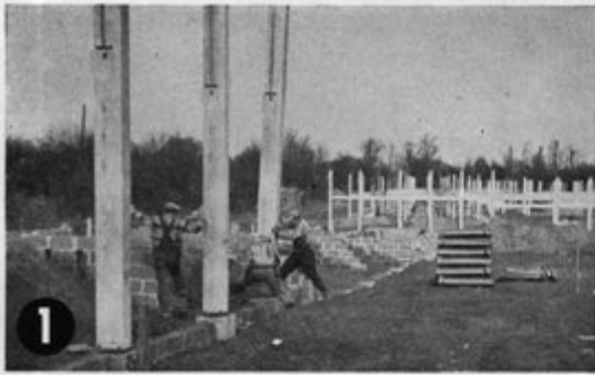
1 First step was to erect the two-story precast concrete columns.
