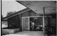
Sunday School classroom. Better light and indoor-outdoor study are advantages of this installation.
