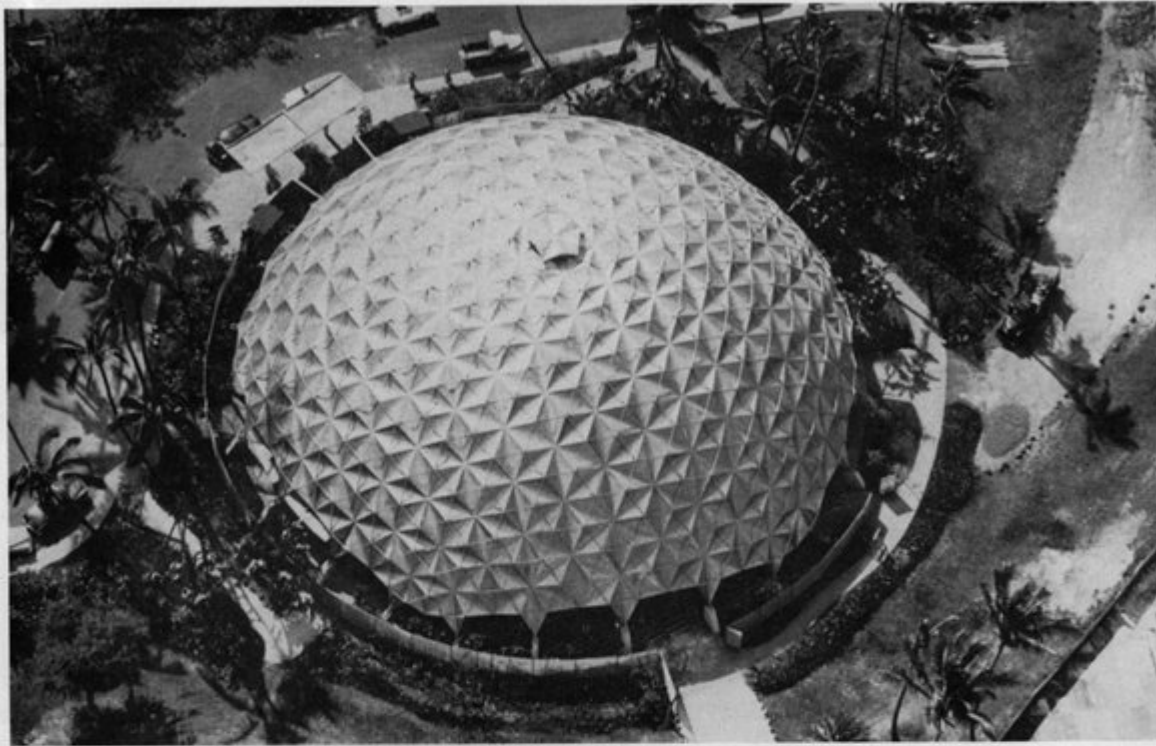
A bird's eye view of a Geodesic Dome designed by Fuller and constructed under license of his patents in Honolulu, during February of this year. It was built to house a convention arena and as a philharmonic concert hall and measures 150 feet in diameter. This dome, fabricated of aluminum by the Kaiser Company was erected in 24 hours. It served as a prototype for another unit erected in August at Virginia Beach for use as a civic auditorium. This is the first all-aluminum dome. Others, like the restaurant dome at Wood's Hole, Mass., have been built with wood struts and a transparent plastic covering.
