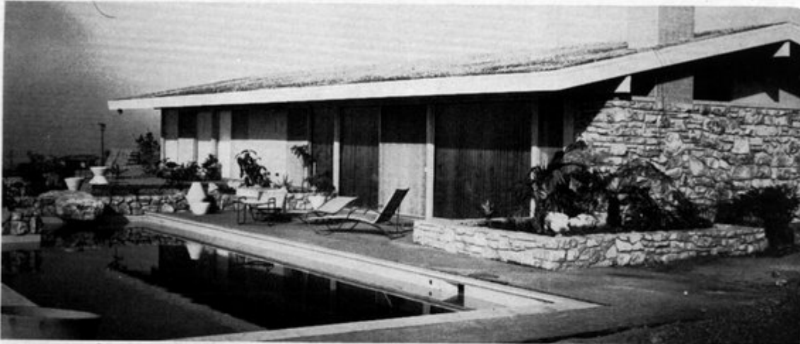
STRONGHOLD and SCREW-TITE Nails were specified exclusively for Research House '56, overlooking the Pacific from above Palos Verdes Drive South, Los Angeles. Architect: Daniel Dworsky, AIA. Builder: Bert Pinckney and Associates.
