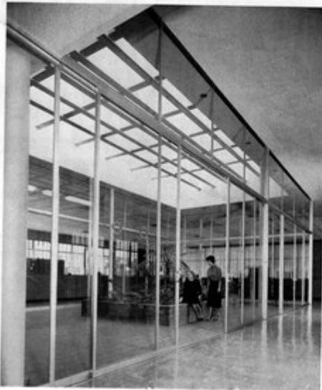
Economical flush threshold is combined with Ador sliding glass doors in pharmacy.
