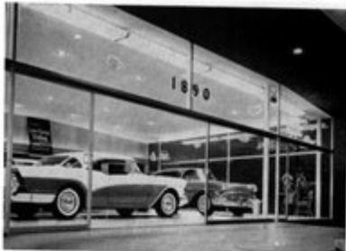
48' wide opening was custom engineered by Ador for this new car showroom.
