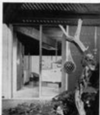
↑ CHEERFUL KITCHEN has wall of floor to ceiling fixed glass at one end and 6' Ador sliding glass door at other end.
