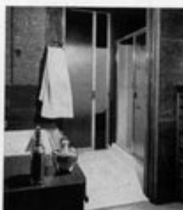
↑ ADJOINING MR. AND MRS. BATHS via 2' Ador doors which slide into wall pockets. Obscure, fluted glass provides privacy.
