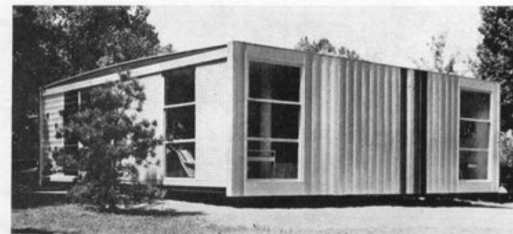
The "pavilion" designed by architect Gio Ponti was actually a small house-apartment, constructed of polychrome vitreous concrete of translucent character and containing an exhibit of furnishings and accessories.
