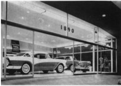
48' wide opening was custom engineered by Ador for this new car showroom.
