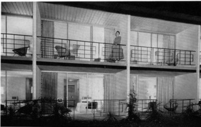
Open display of inviting room interiors is a strong competitive advantage to this motel with Ador sliding glass doors.
