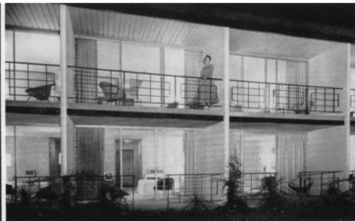
Open display of inviting room interiors is a strong competitive advantage in this motel with Ader sliding glass doors.
