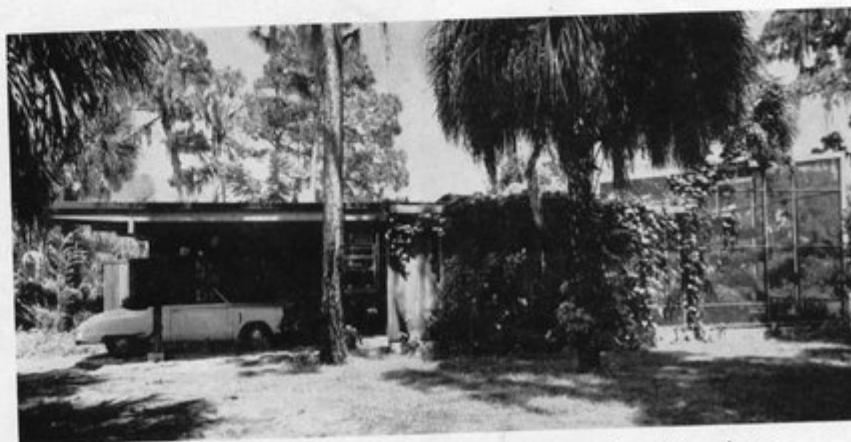
Carport serves as entrance shelter to both front (through porch) and rear entrances. Screen cage over patio was made high to enhance outdoor effect.
