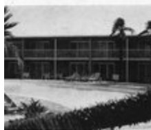
Free access of guests to pool and patio is assured by get-up operation of Ader doors. Open view adds safe luxury.
