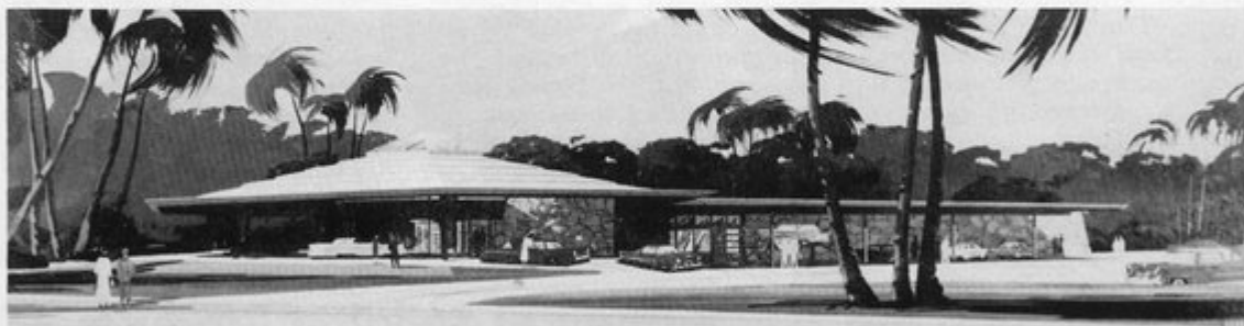
Carlisle-Porter, Lincoln Mercury Motor Co., Clearwater, Fla. Rilco Hip Beams, 5 1/4"x26"x39'1" to 52'8" long. Also purlins & facias. Rilco Deck of Western Red Cedar. Architect, John Randal McDonald.
