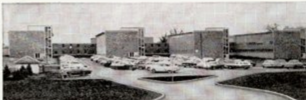
12,200 square feet of Porcelo Panels were used in the construction of the New Engineering Buildings at Colorado A. & M. College.
