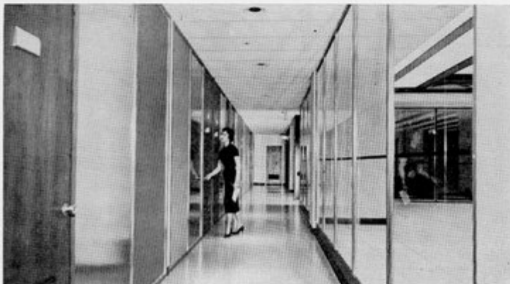
A wide variety of paneling material can be utilized for Unistrut partitions.
