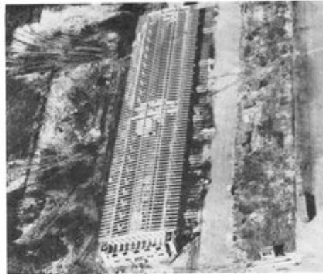
This view of a new building under construction shows interesting pattern formed by prestressed concrete joists before roof deck was placed.
