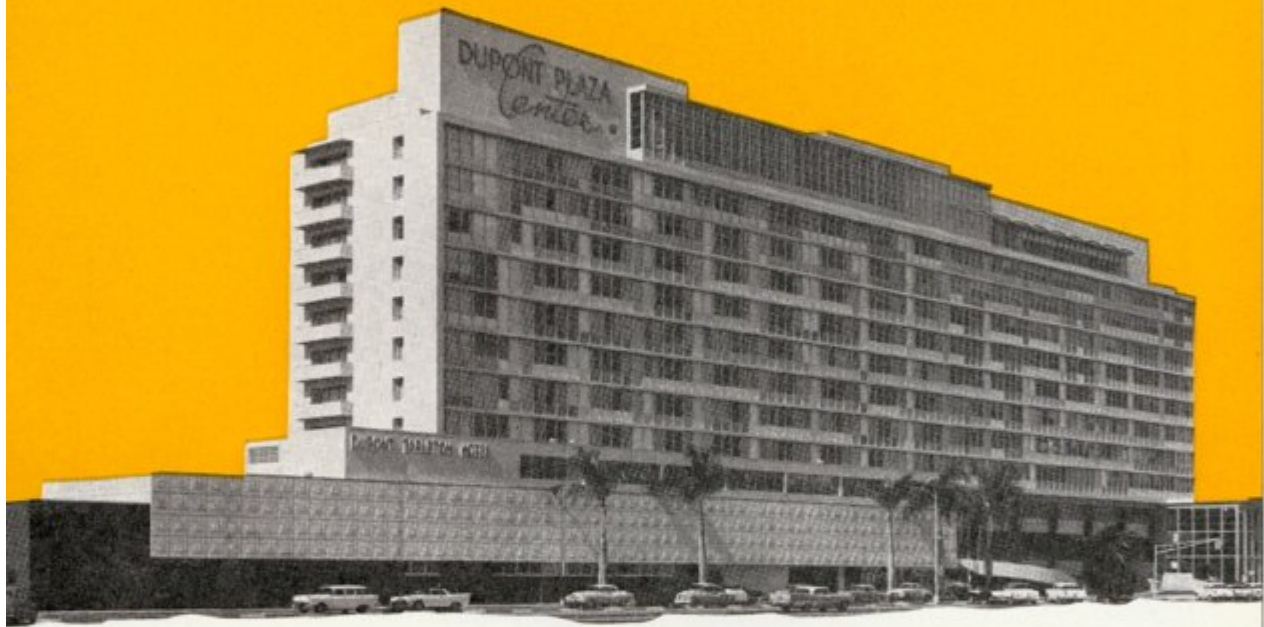
Dupont Plaza Center, John E. Petersen (1903-1957), Frank H. Shuffin, AIA, architects, Arkin Construction Co., general contractors, was faced with Florida Oolite Limestone by Kermit V. Miller
