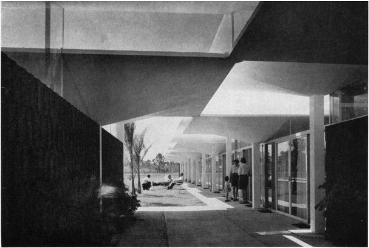
Above, juncture of two wings of what will ultimately become a U-shaped plan provides a sheltered court, sheltered by the half-shells of the precast concrete units which form both framing and roof members. Note how the structure is scaled to human dimensions, yet conveys an impression of soaring height.
