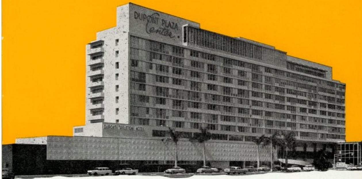
Dupont Plaza Center, John E. Petersen (1903-1957), Frank H. Shufflin, AIA, architects, Arkin Construction Co., general contractors, was faced with Florida Oolite Limestone by Kermit V. Miller
