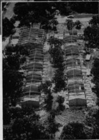
Rilco pitched beams, 36', 40', 56' long, spaced 10' o.c. Rilco western red Cedar Deck serves as ceiling, decoration and insulation.
