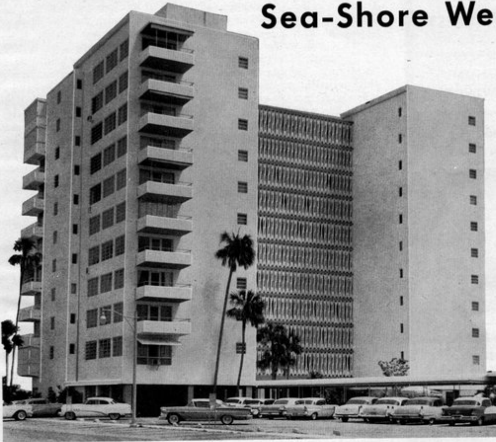
Exterior of the Springtide Coop Apartments at Ft. Lauderdale, Florida, Polevitsky & Johnson, architects, has been coated with Evershield Liquid Tile over cement stucco and concrete block surfaces.
