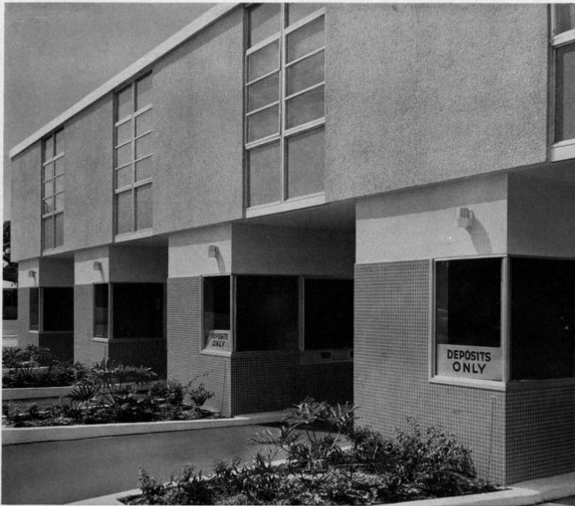
Scored Tile in Design SD-1, applied to Drive-in Tellers' Booths of the new Merchants Bank Building, Miami. Architect: Montgomery Atwater. Builder: Witters Construction Company. Tile Contractor: Manze Tile Company, Inc.
