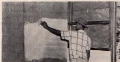
Above photo shows ease of finishing IRB panels. Finishing procedure is the same as with regular Par-WOOD and Par-TEX panels.
